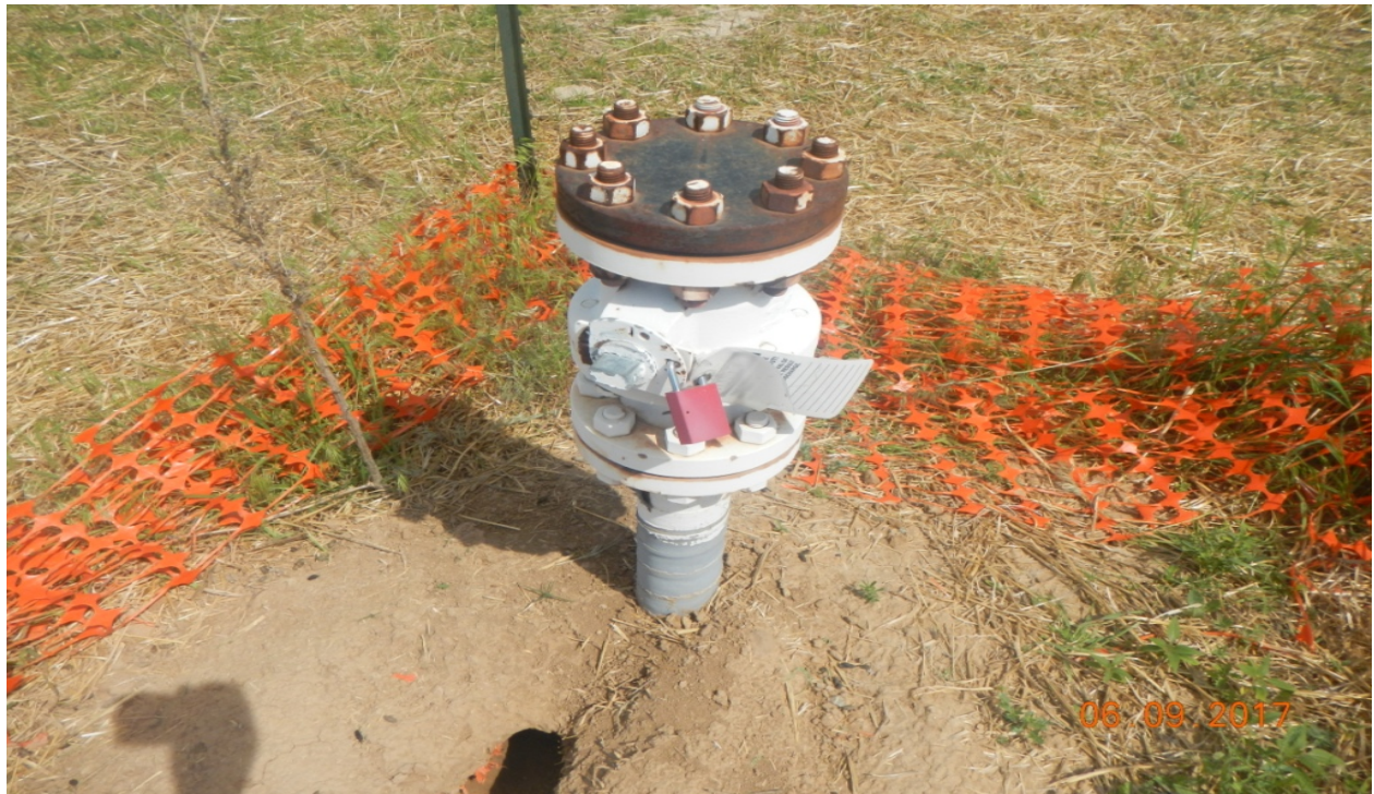
photo 5: The pipe riser has been locked and tagged out.
