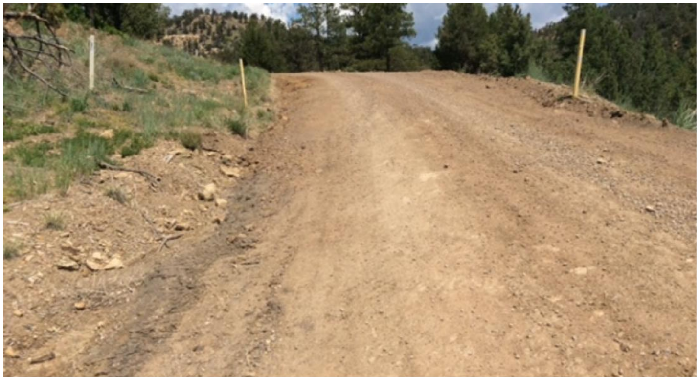
Photo 2: The main road surface has been bladed and crowned to correct the erosion issues.
