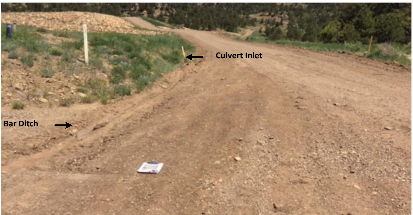
Photo 4: The bar ditch was dominated to direct run off to the down gradient culvert inlet.
