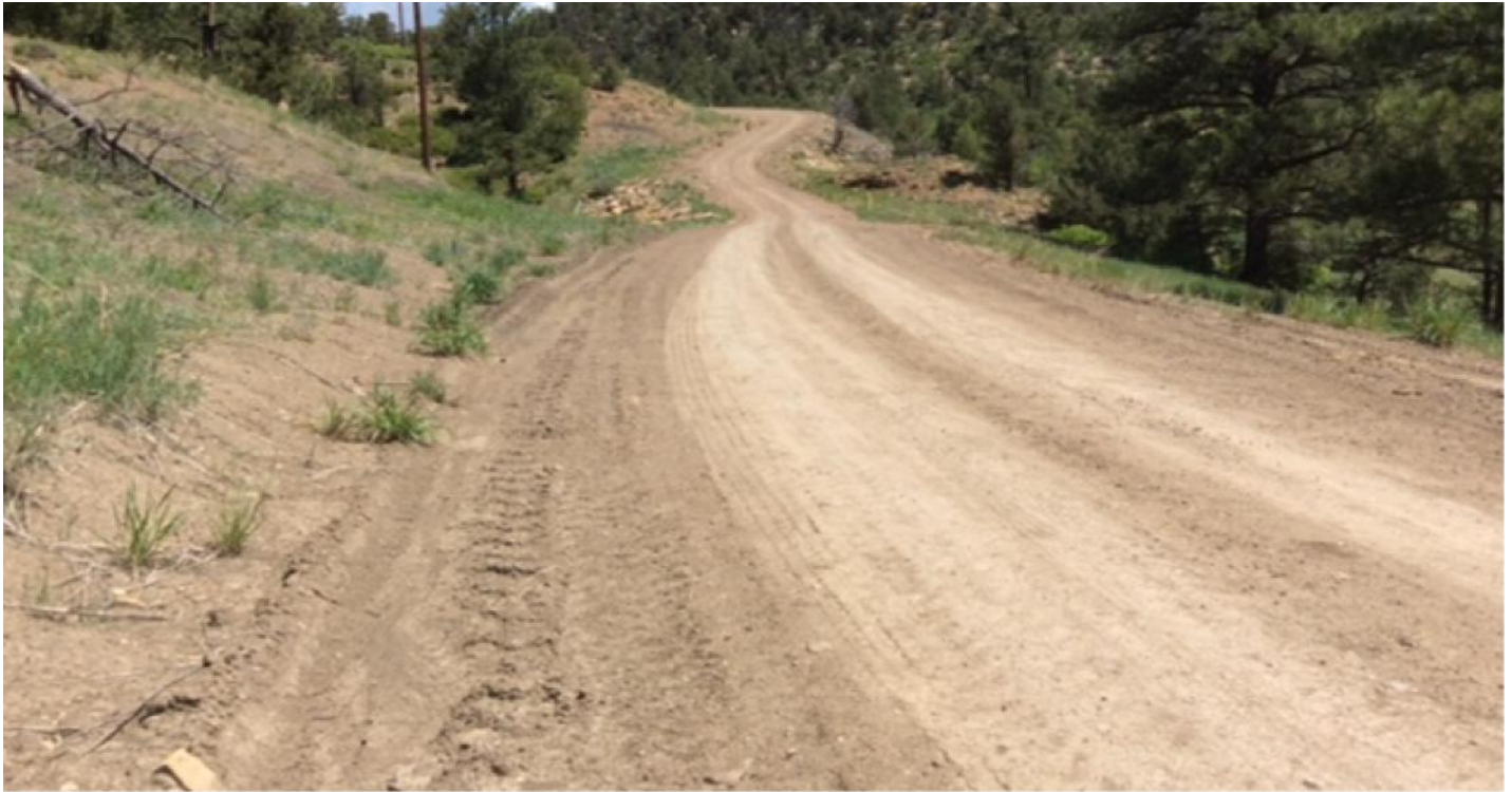
Photo 1: Facing northeast along the main access road. Bladed the roadway and crowned the driving surface to establish sheet flow.
