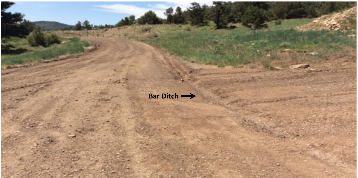
Photo 3: Facing south toward the well pad access road. Gravel was pulled into the access road and surface crowned to create sheet flow. The bar ditch was dominated to direct run off to the down gradient culvert inlet, to control erosion of the main access road.
