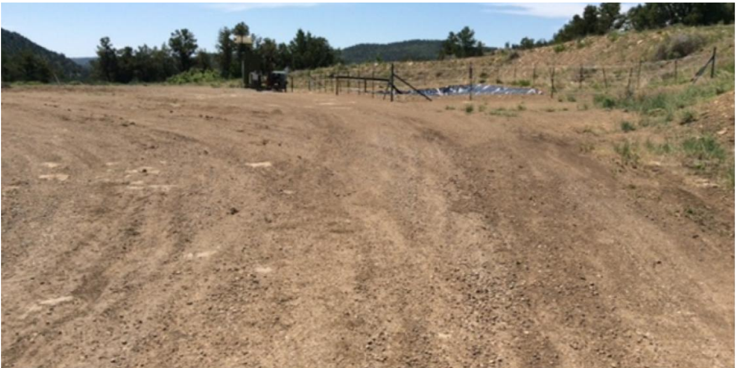
Photo 6: Facing south toward location. Pulled gravel onto the driving surface and bladed tire ruts.
