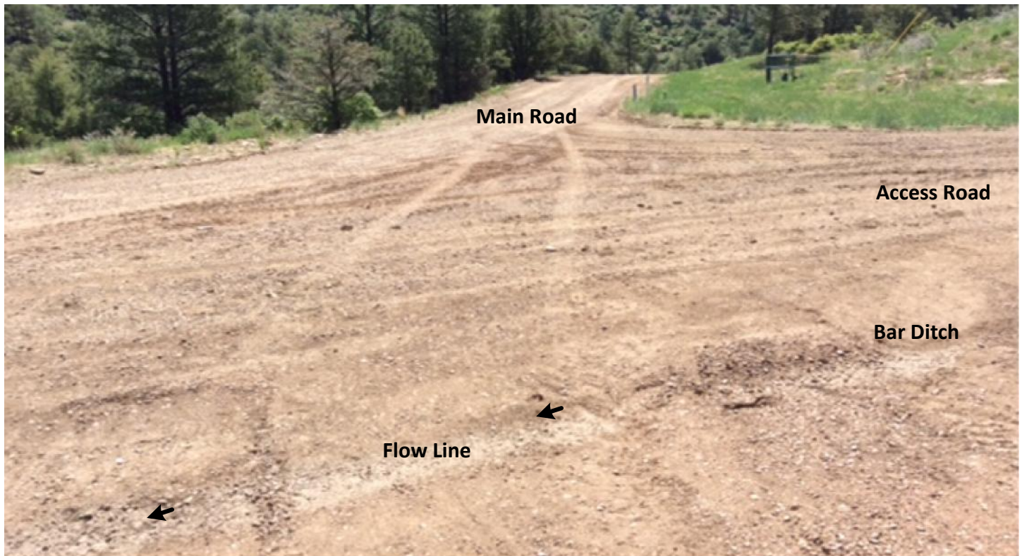
Photo 5: Intersection of main Lopez road and GE 21-15X access road. Pulled gravel onto the driving surface and re-established the bar ditch.
