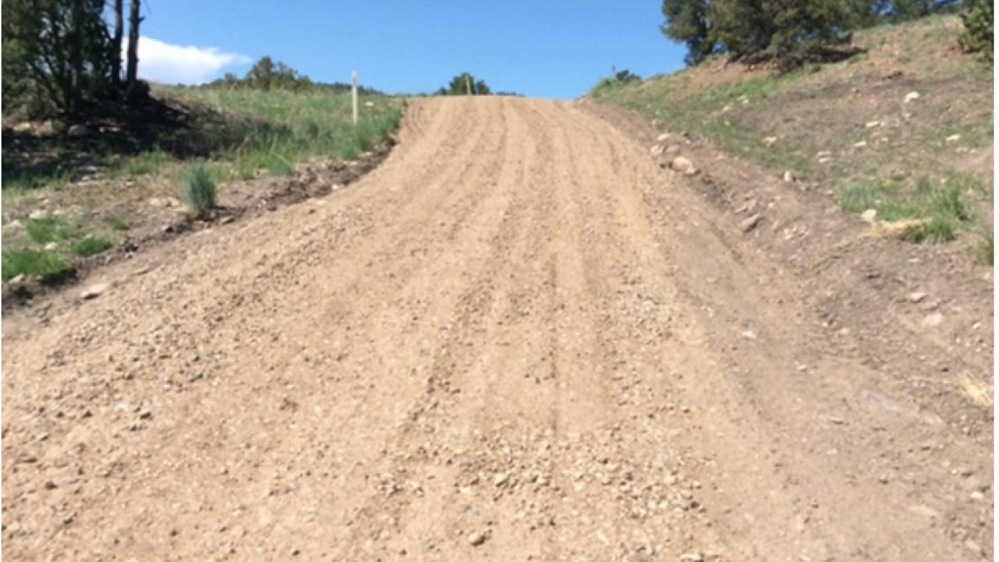
Photo 1: Facing southwest along the access road. Installed gravel and crowned the driving surface to establish sheet flow.
