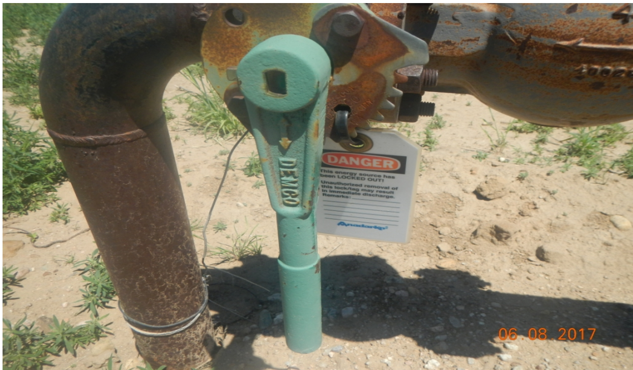
photo 4: Tag out has been applied to this valve at the pipe riser.
