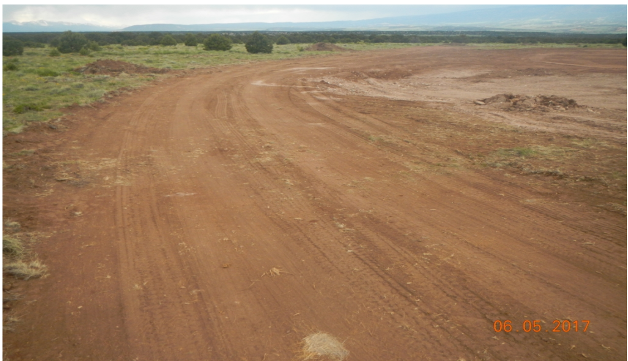
photo 4: Facing northwest along the access road. No stormwater perimeter controls are present.
