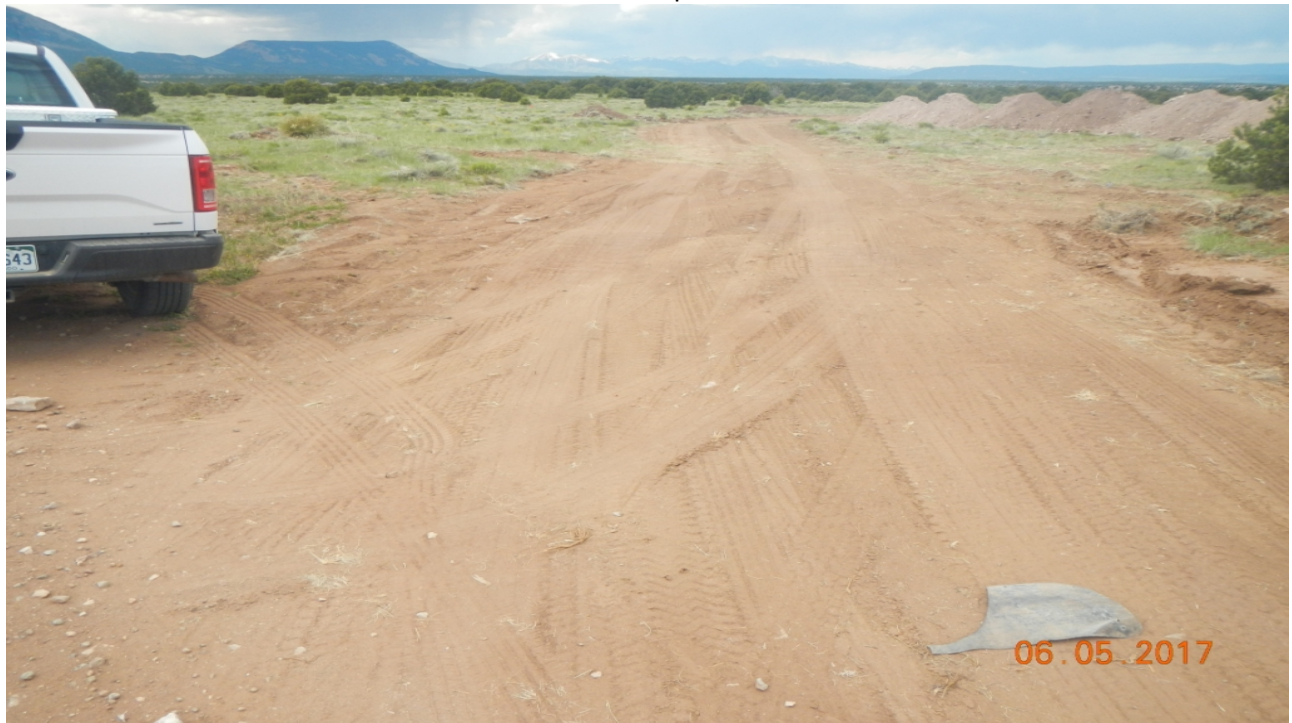
photo 2: Facing northwest toward recently constructed access road off of county road 530. There is no vehicle tracking controls in place.
