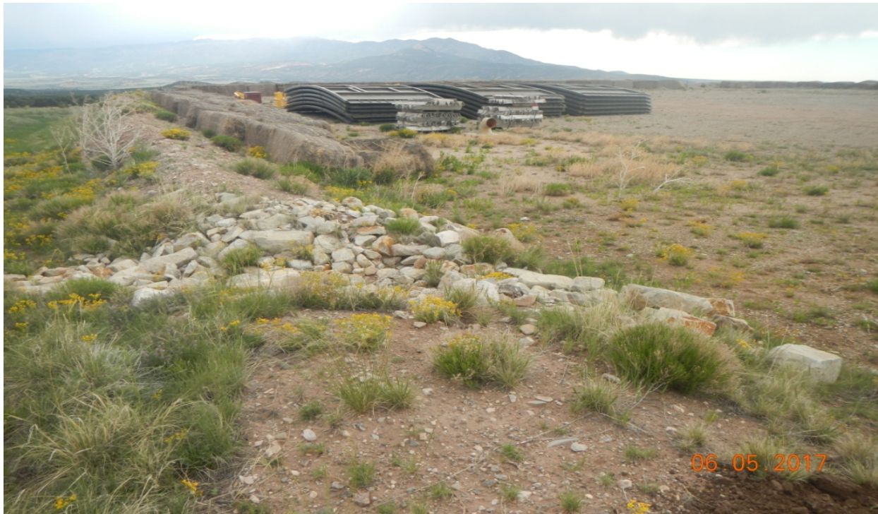
photo 9: West side of the location facing north toward unused equipment. There is rock rip/rap BMP in place for stormwater outlet.
