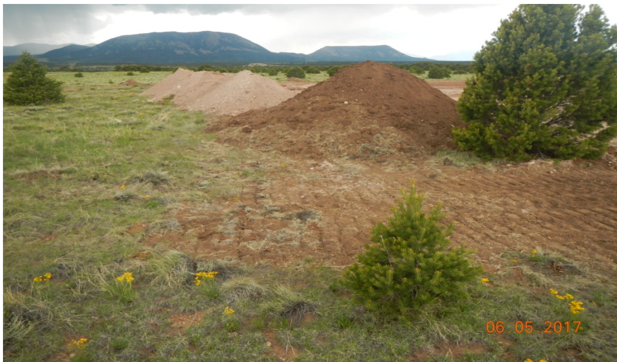
photo 6: Southeast side facing west toward soil piles. No stormwater perimeter controls are present and soil stockpiles are not stabilized.
