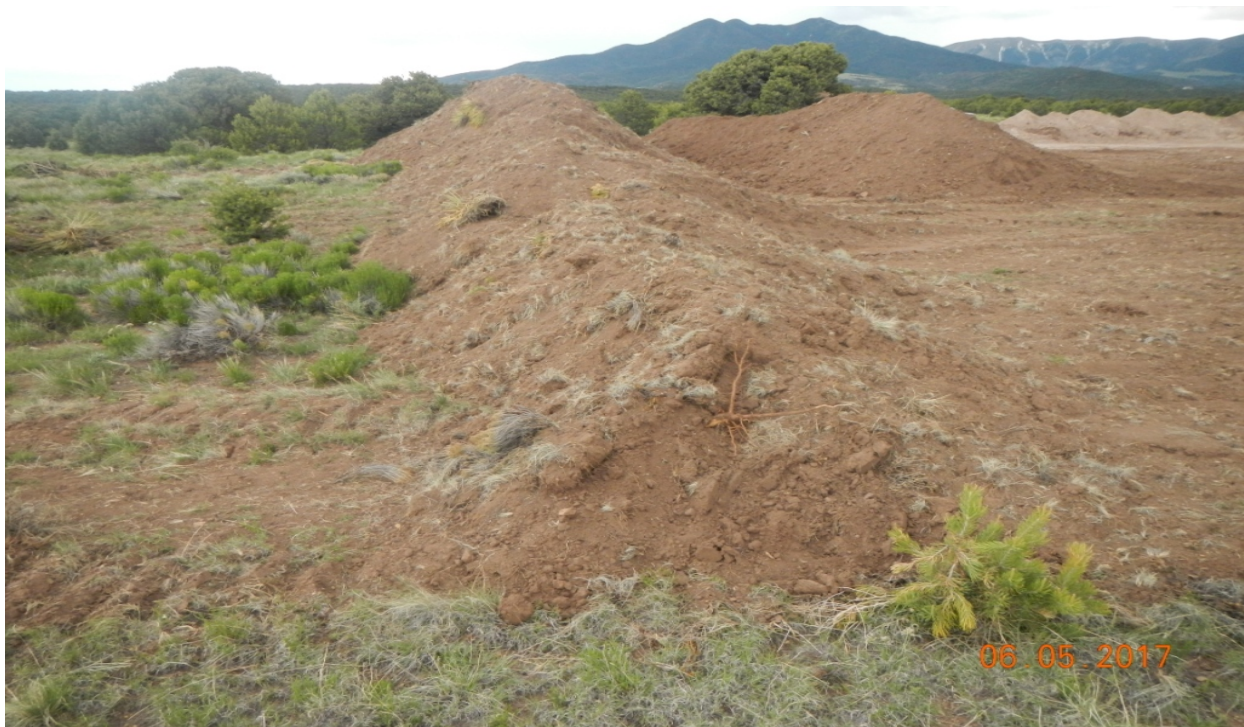
photo 8: Northeast side facing south toward the topsoil piles. No stormwater perimeter controls are present and soil stockpiles are not stabilized.
