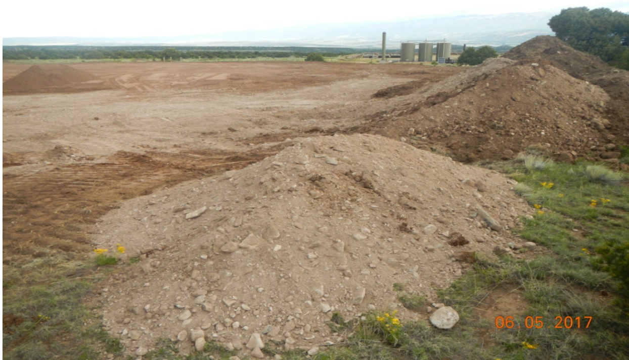
photo 7: Southeast side facing northwest. No stormwater perimeter controls are present and soil stockpiles are not stabilized.
