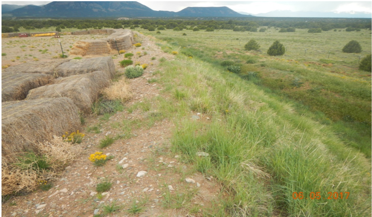
photo 7: North side of the location facing west. There is a stormwater berm around the northern perimeter of the location.
