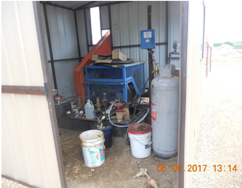
Fittings and bucket in engine shed. Note stained soil as well
