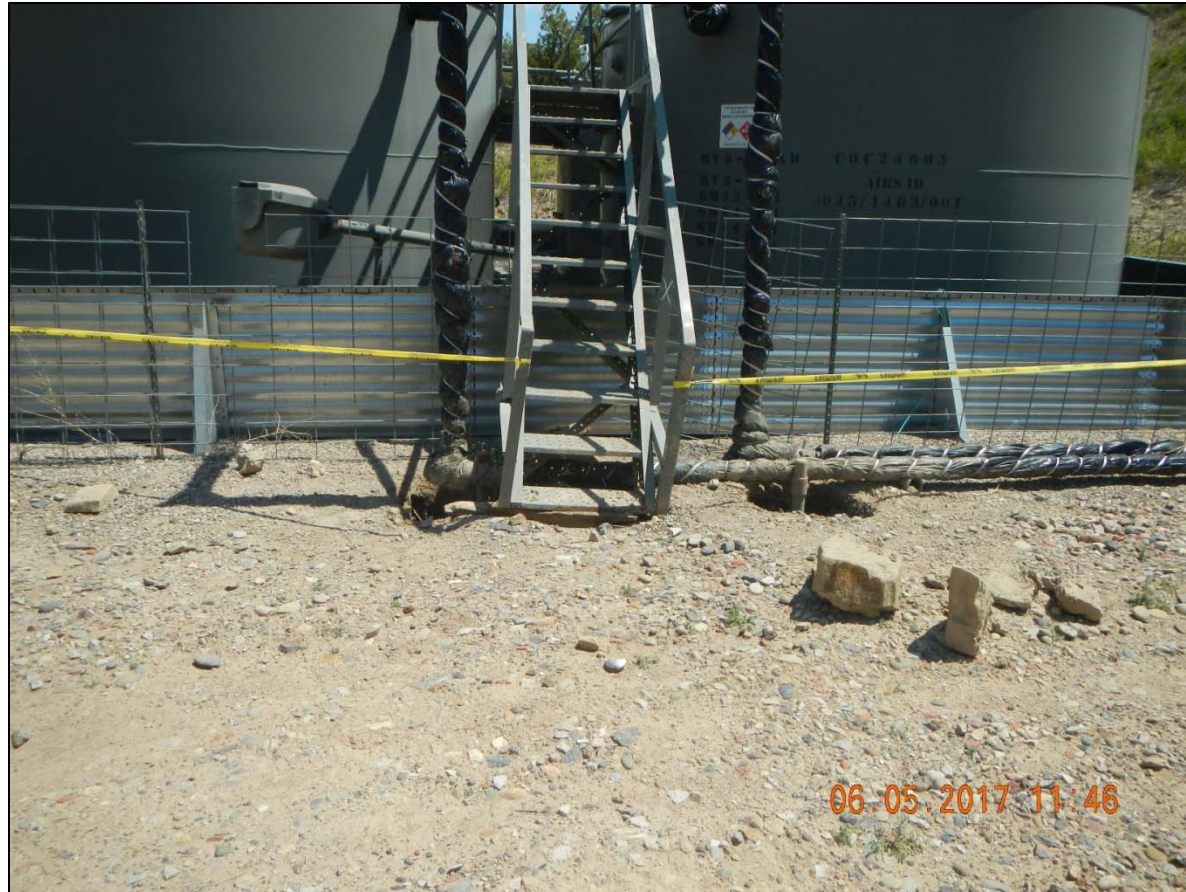
Tank battery: Potholes around flowlines not in use.
