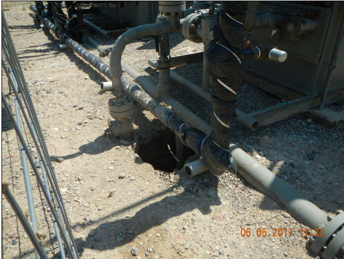
Separators: Potholes around flowlines not in use.
