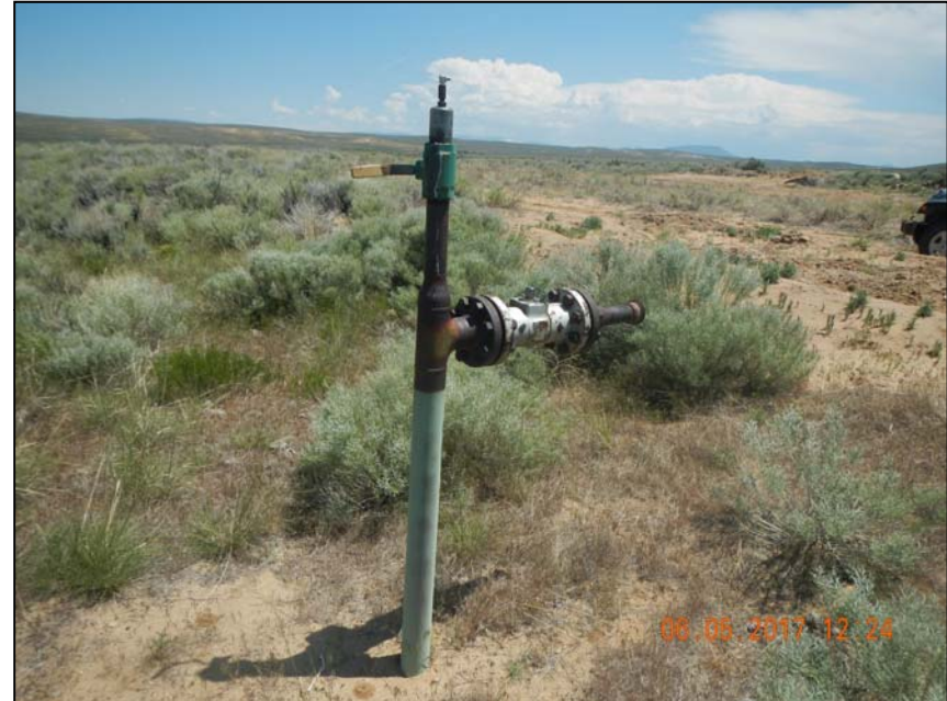
Photo 4. Unmarked 3" steel riser at 40.97712, -107.62637.
