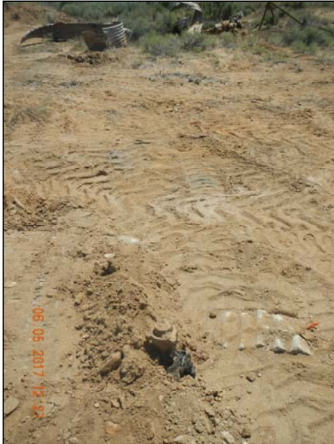
Photo 3. Unmarked 2" steel riser at 40.97718, -107.62582.
