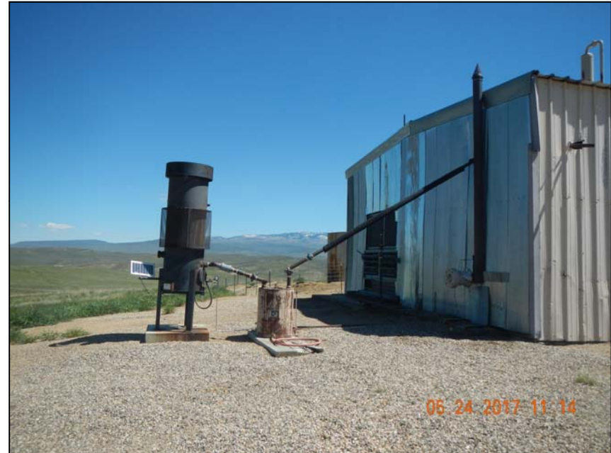
Photo 6. Compressor and ECD with flowlines.
