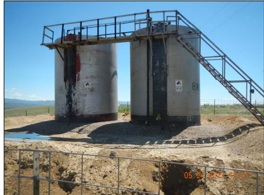
Photo 8. Tank battery with animal burrows visible in berm.
