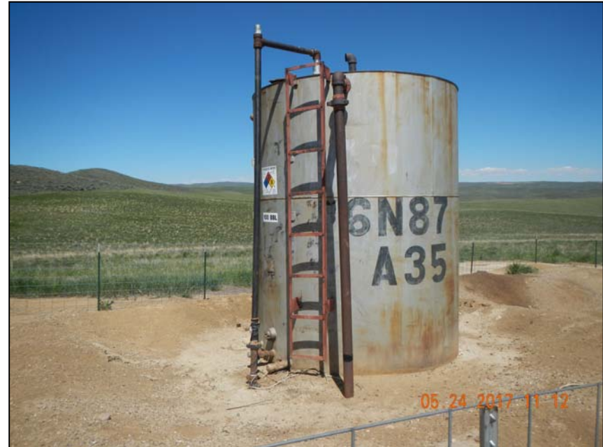
Photo 4. Produced water tank with risers.
