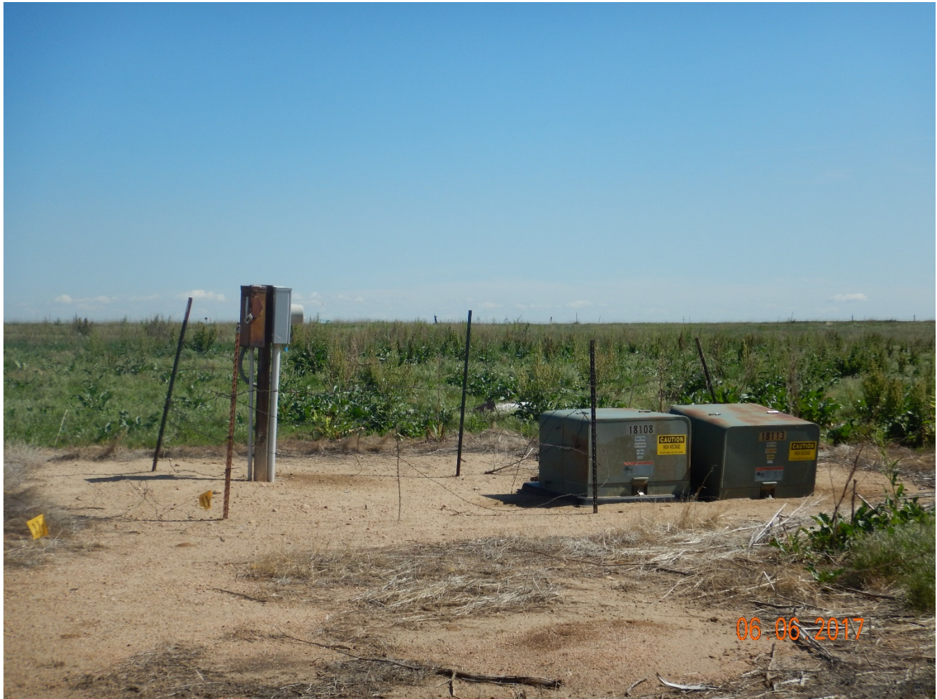
Photo 8 - Electrical control box and transformers NE of pumping unit. Note: barbed wire fence in need of repair.
