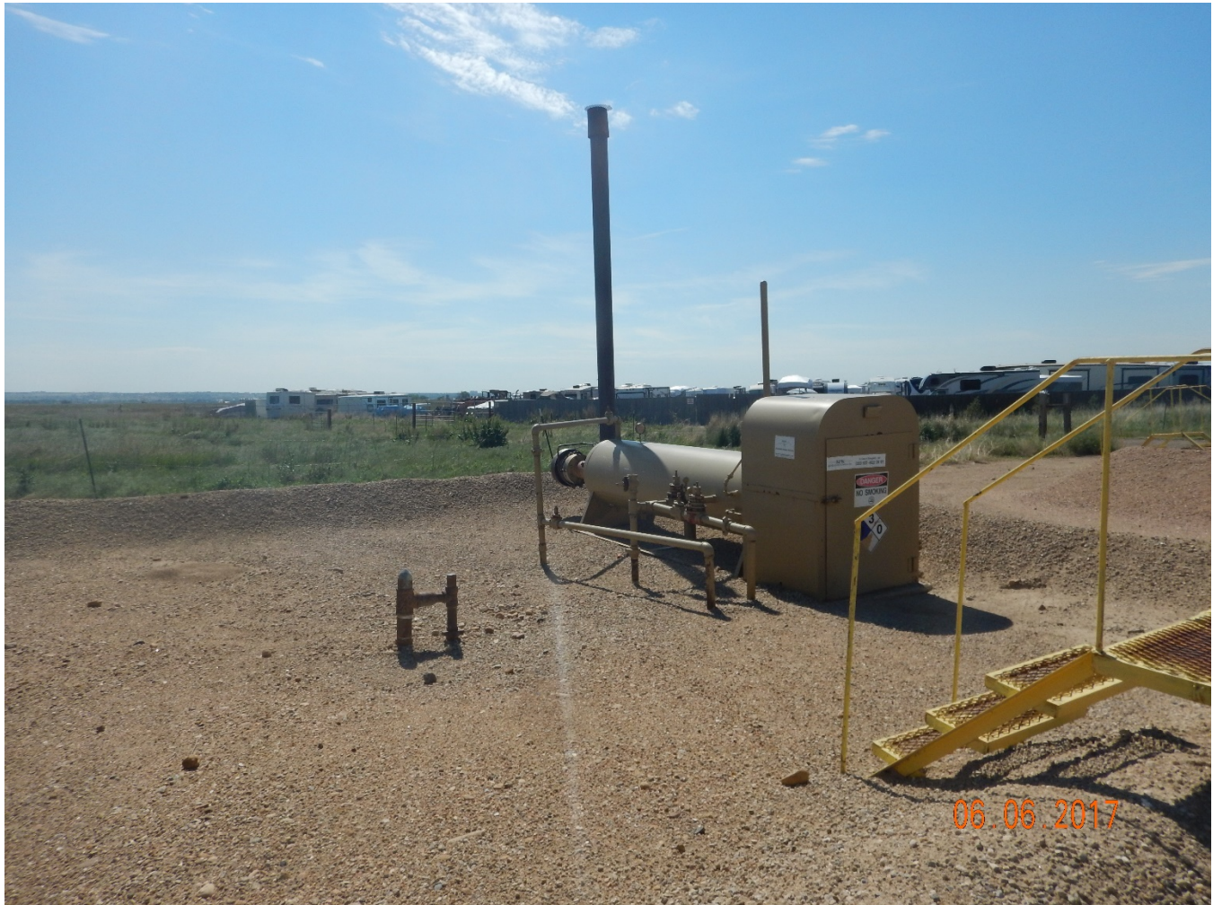
Photo 13 - Flowline risers at horizontal separators may be out of compliance with 2017 Flowline NTO.
