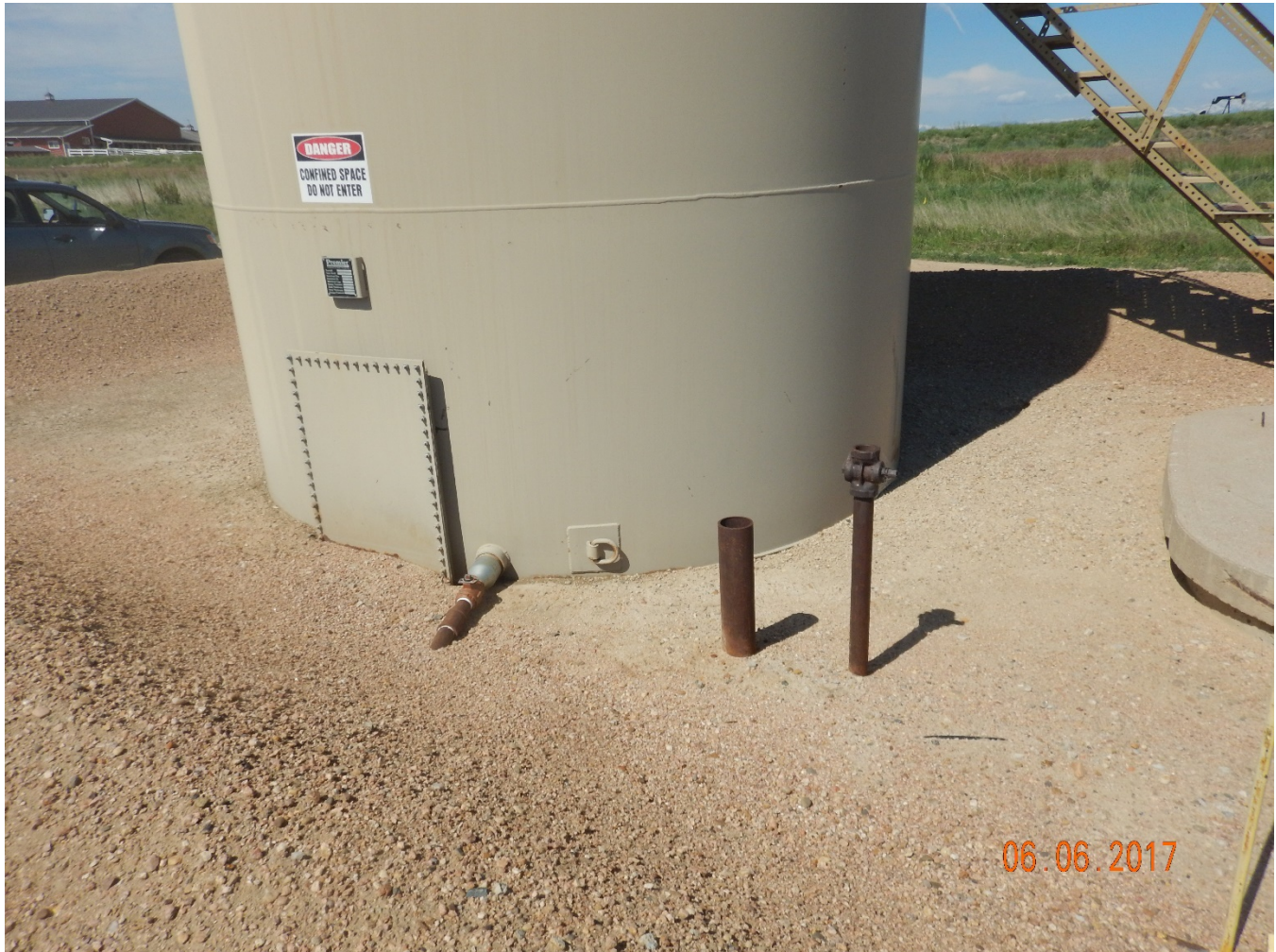
Photo 10 - Flowline risers NE of tank battery are out of compliance with 2017 Flowline NTO.
