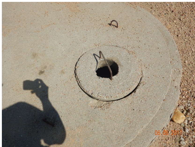
Photos 11 & 12 - Produced water vault is open to the atmosphere.
