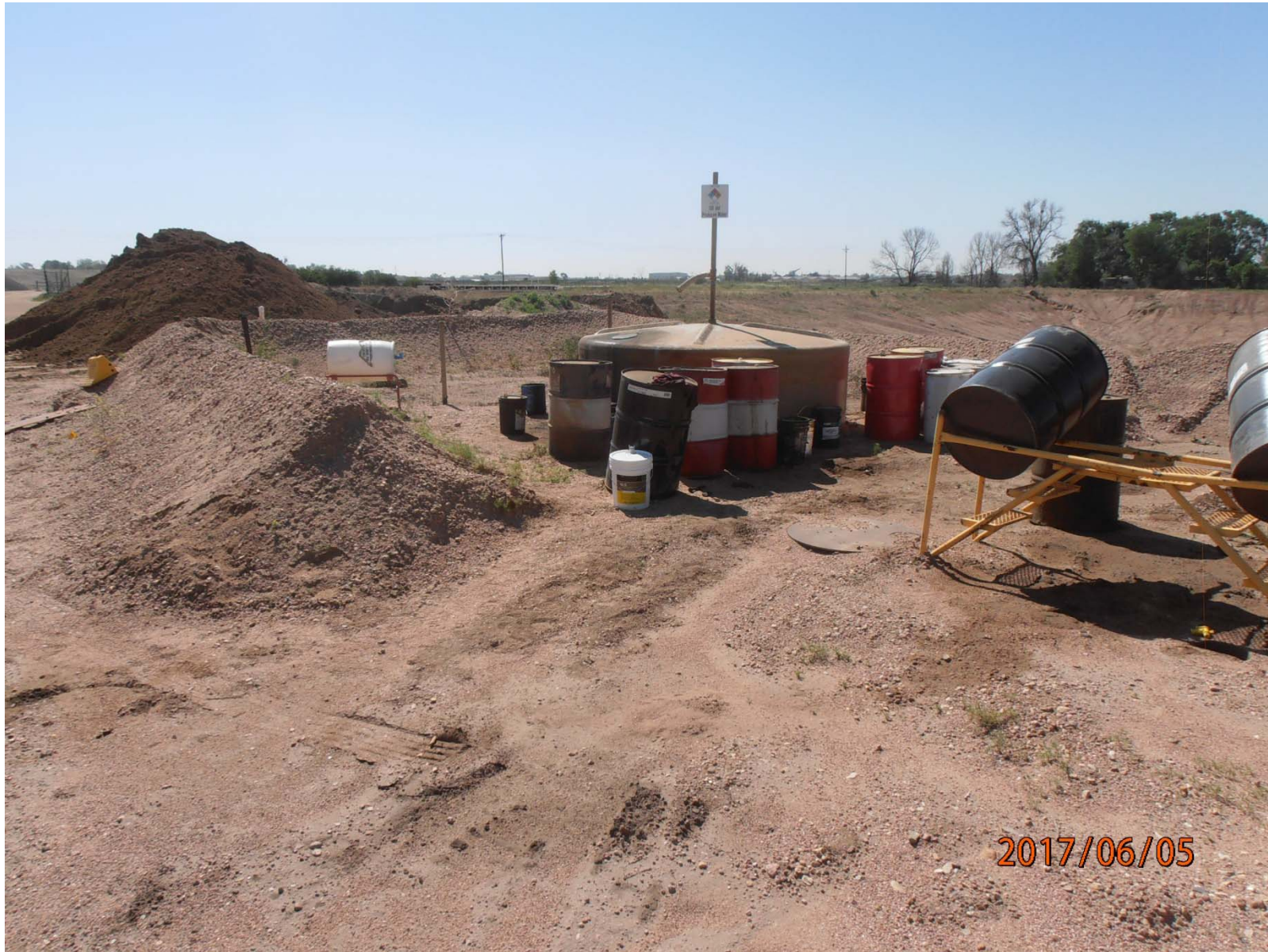
Former production facility showing risers for product piping and remaining partially buried fiberglass produced water vessel. Looking southeast.
