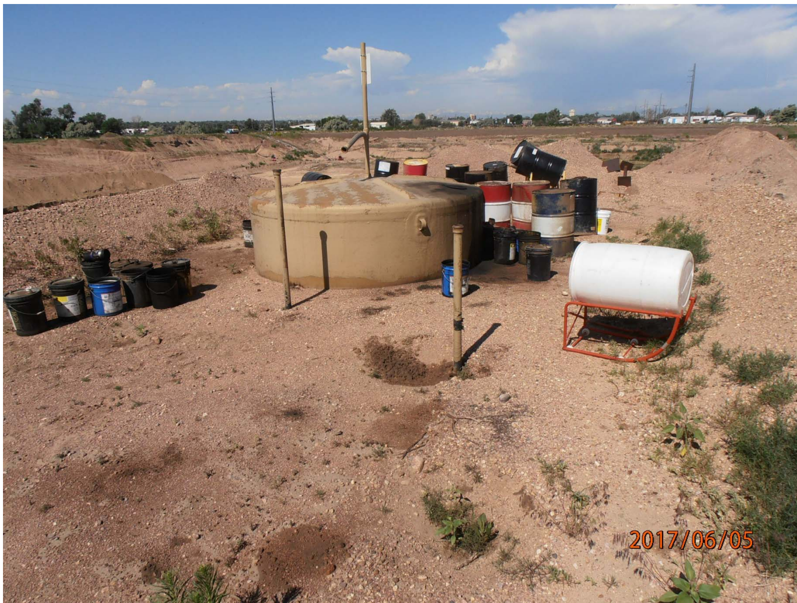
Former production facility showing risers for product piping and remaining partially buried fiberglass produced water vessel. Standing in northeast corner of containment looking west.
