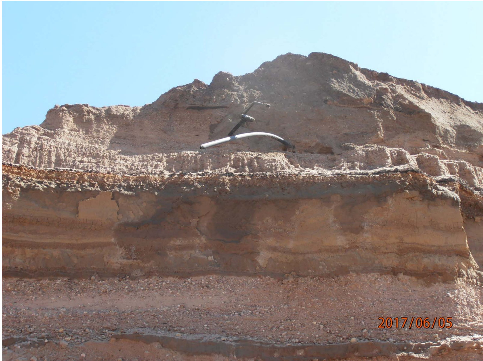
Flowlines protruding from gravel pit wall. COGCC unable to inspect sand near flowline due to safety hazard of steep excavation wall.
