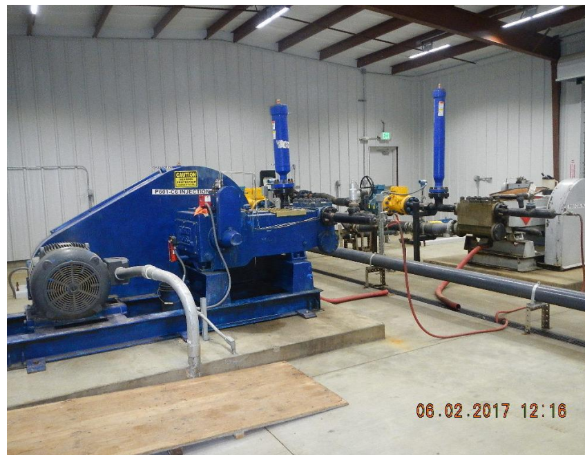
Photo 2 Prime movers inside pump house 1-175 HP and 1-165 HP
