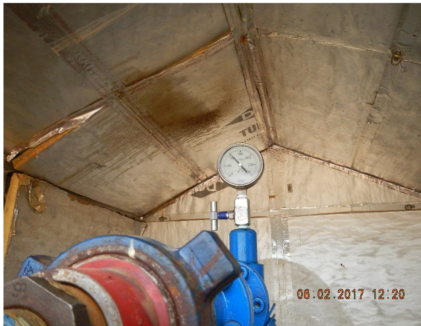
Photo 5 Inj Tubing pressure gauge 800 PSI
