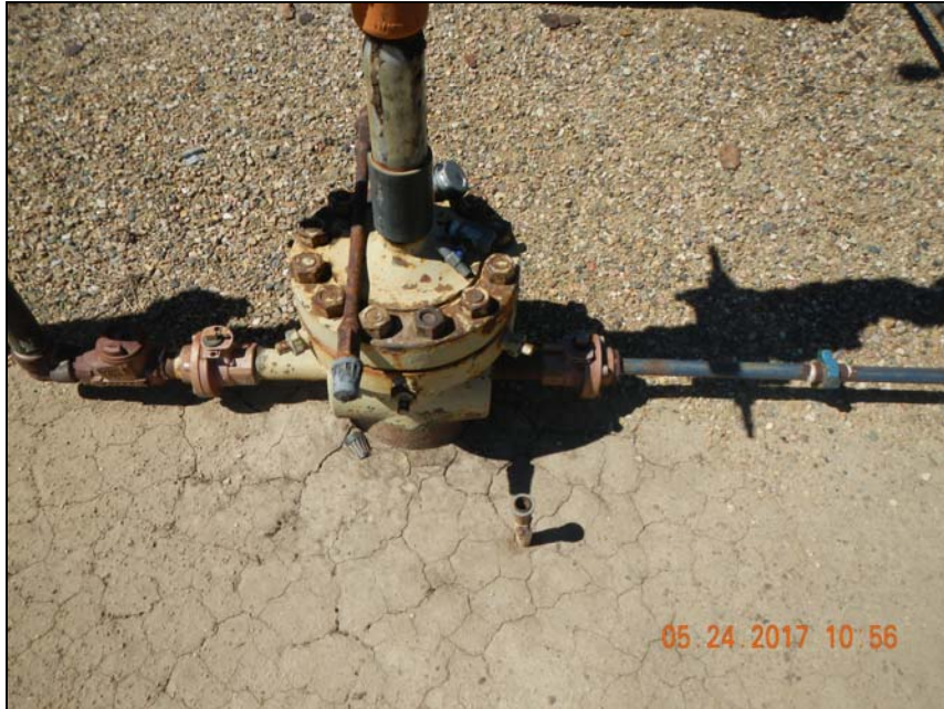
Photo 3. 1 -1" steel riser not in use at wellhead.
