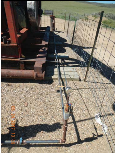
Photo 5. 1' steel line running to separator.
