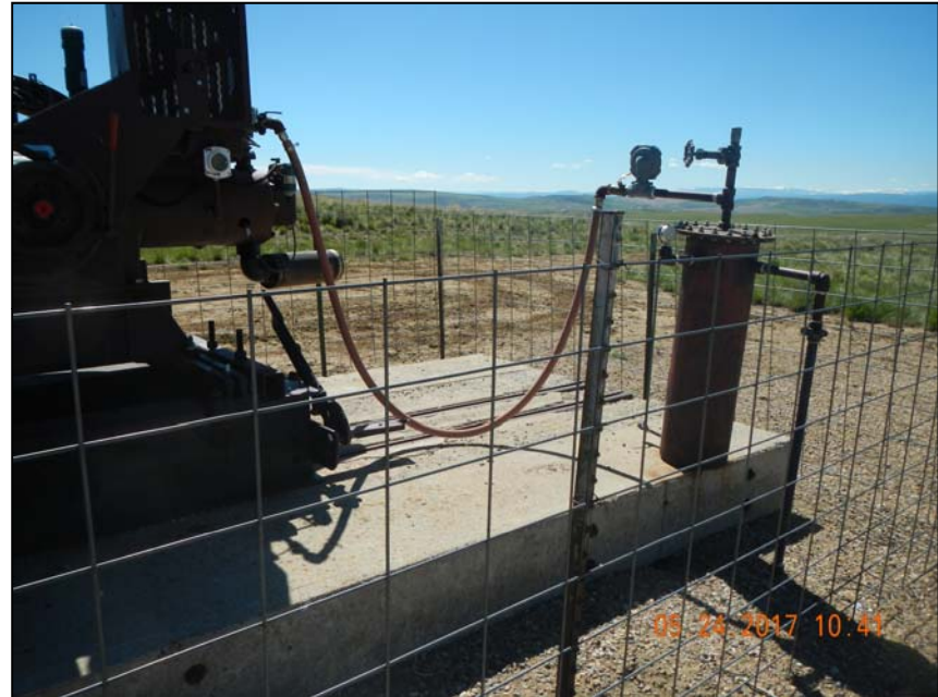
Photo 6. Lines connecting separator and motor.
