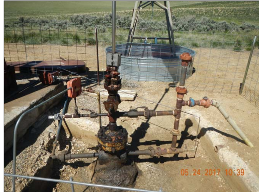
Photo 4. Wellhead assembly with 1 -2" steel riser in use, methanol lines, 1 - 1" steel riser not in use.
