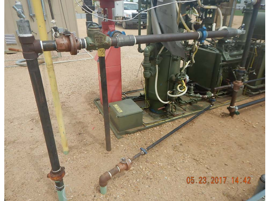
Photo 6: Risers at compressor
