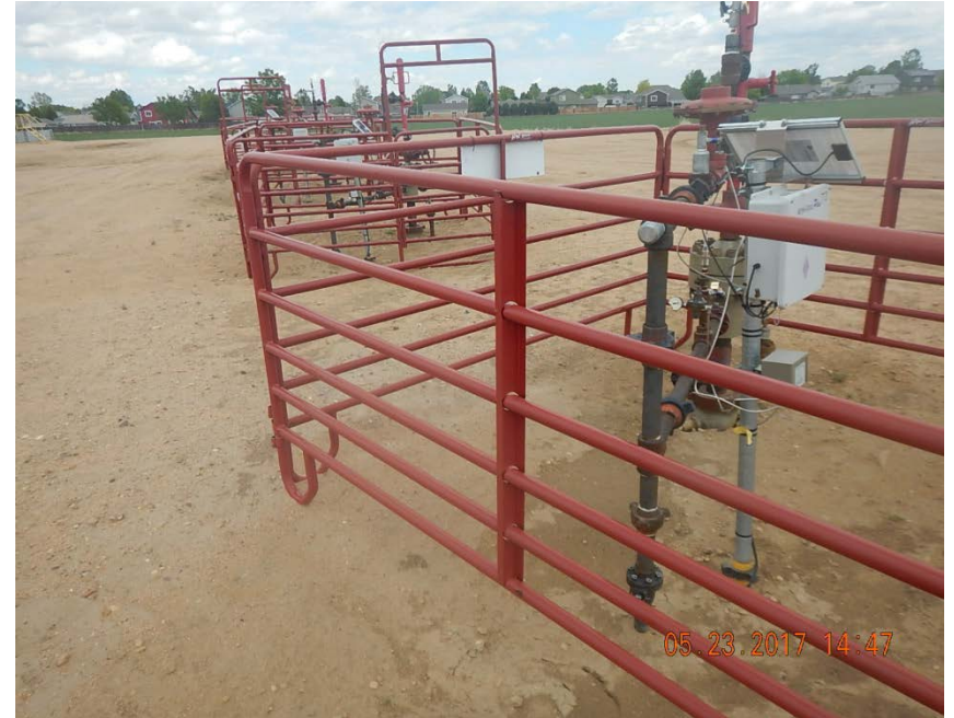
Photo 2: flowlines at wellheads
