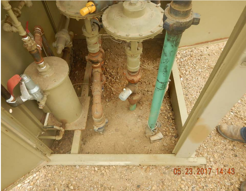
Photo 3: Flowlines in separator house
