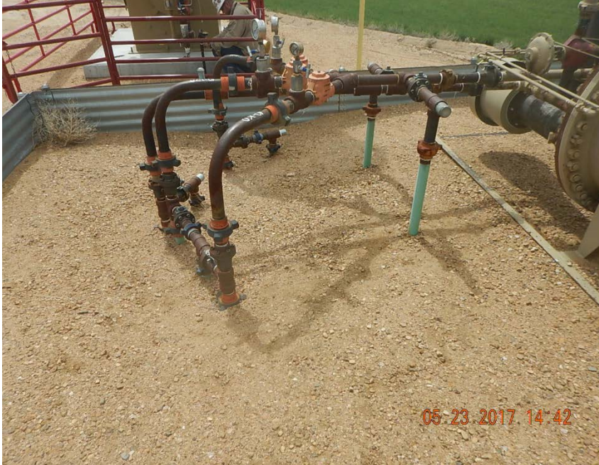
Photo 5: Risers at separator
