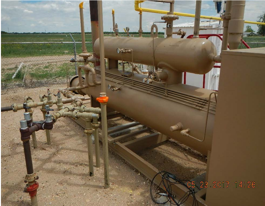
Separator inlet lines N40.32746 W-104.83070
