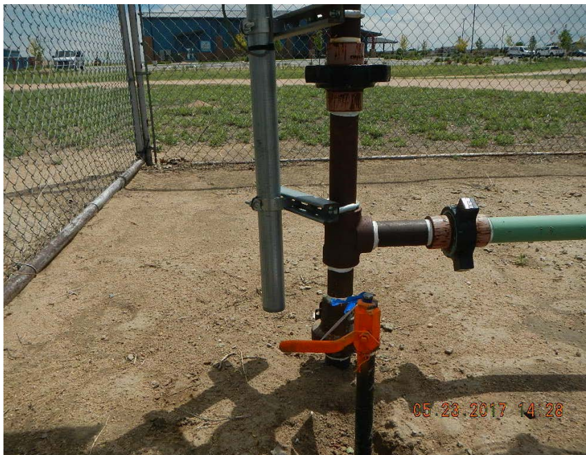
Wellhead flow line risers
