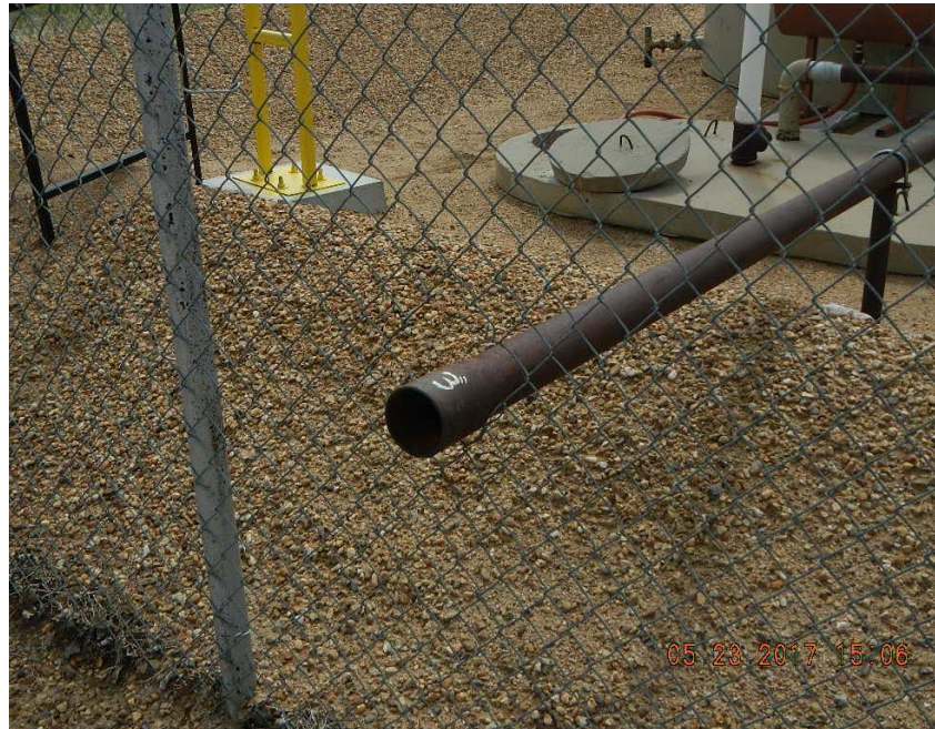
Produced water vault load line
