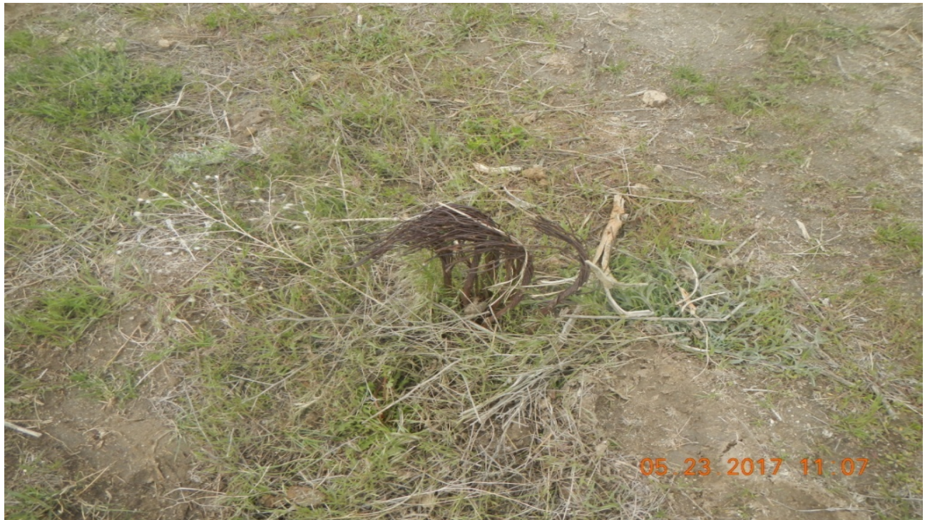
photo 3: A cable was found extending out of the ground which was cut off below ground during this inspection.
