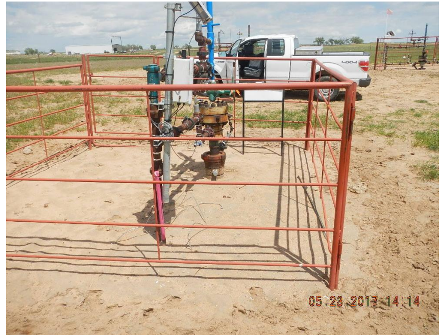
Wellhead with marked and capped flowline from west
