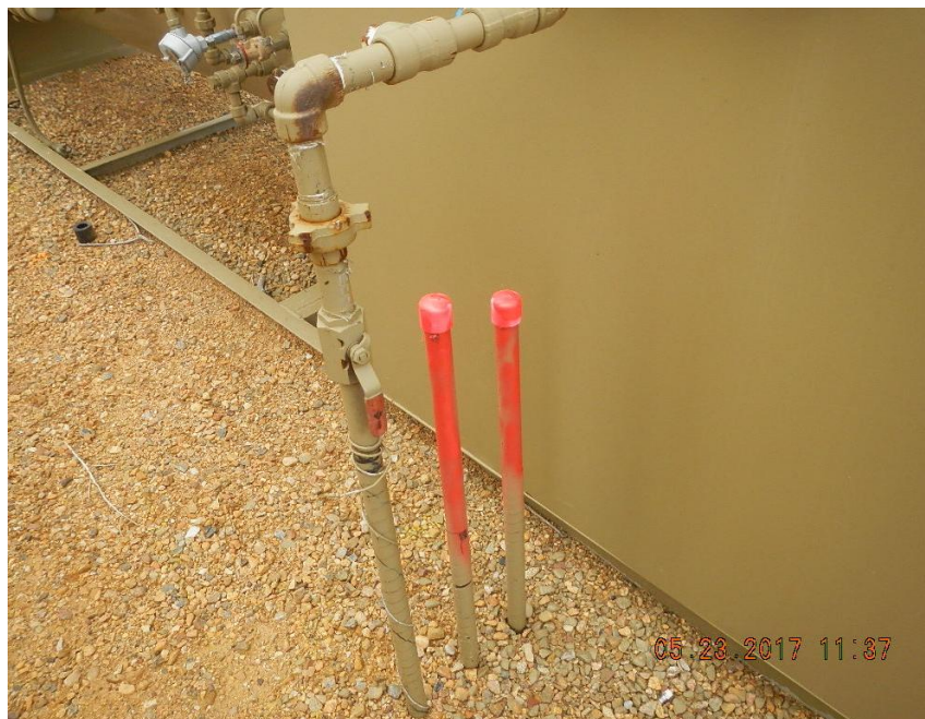
Painted and capped risers (2X) north side of Hartell separator, 40.20676, -104.75459
