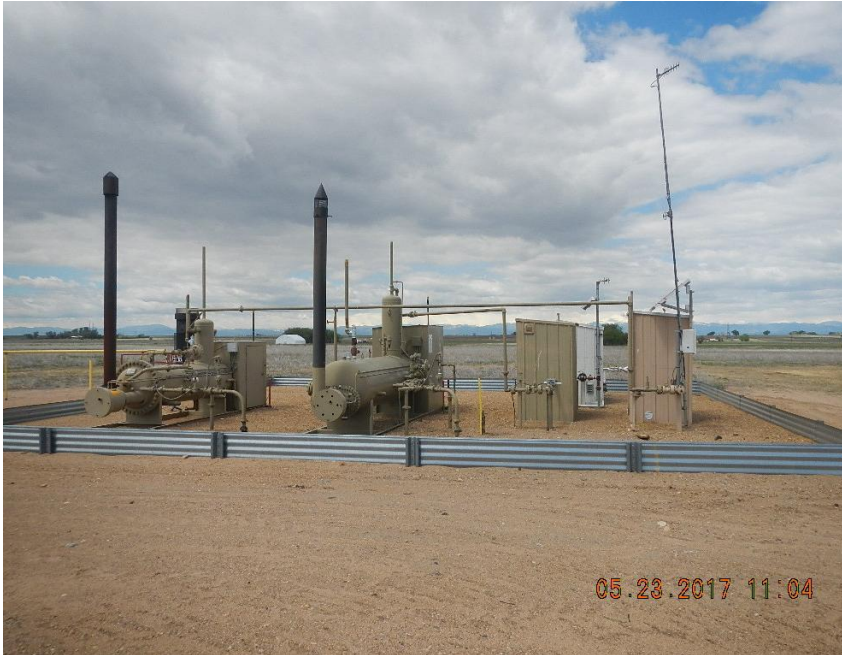
Separators and meter runs from northeast
