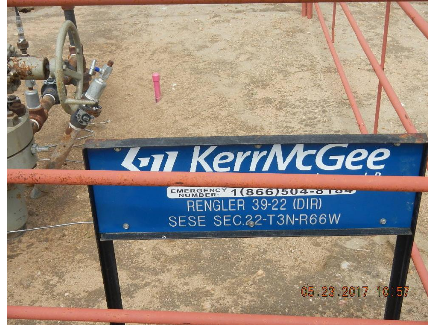
Painted and capped flowline riser at Rengler 39-22 wellhead
