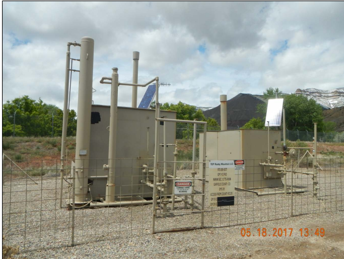
Separators and flow lines
