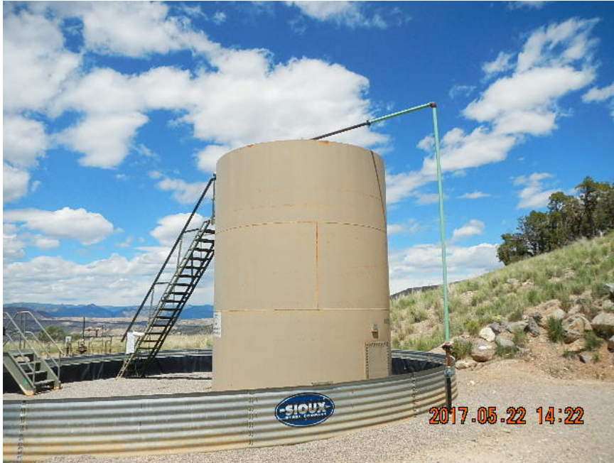
1-2" steel water/oil dump line from separator to tank
