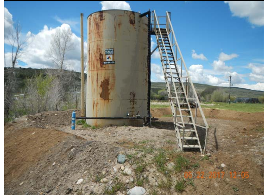
Photo 3. 2 – 2" insulated risers at tank. NFPA diamond still only for produced water.
