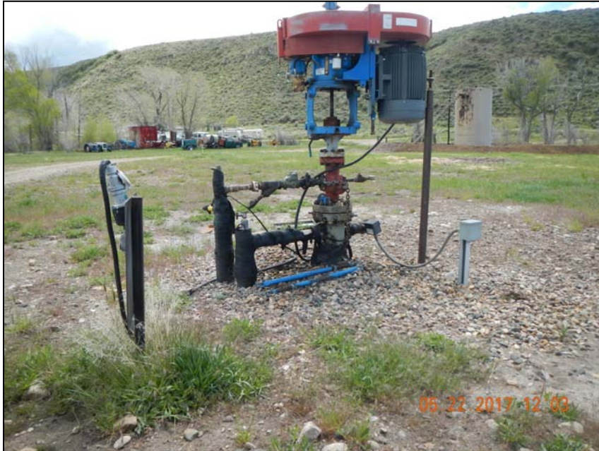
Photo 2. 2 -2" insulated risers at wellhead.
