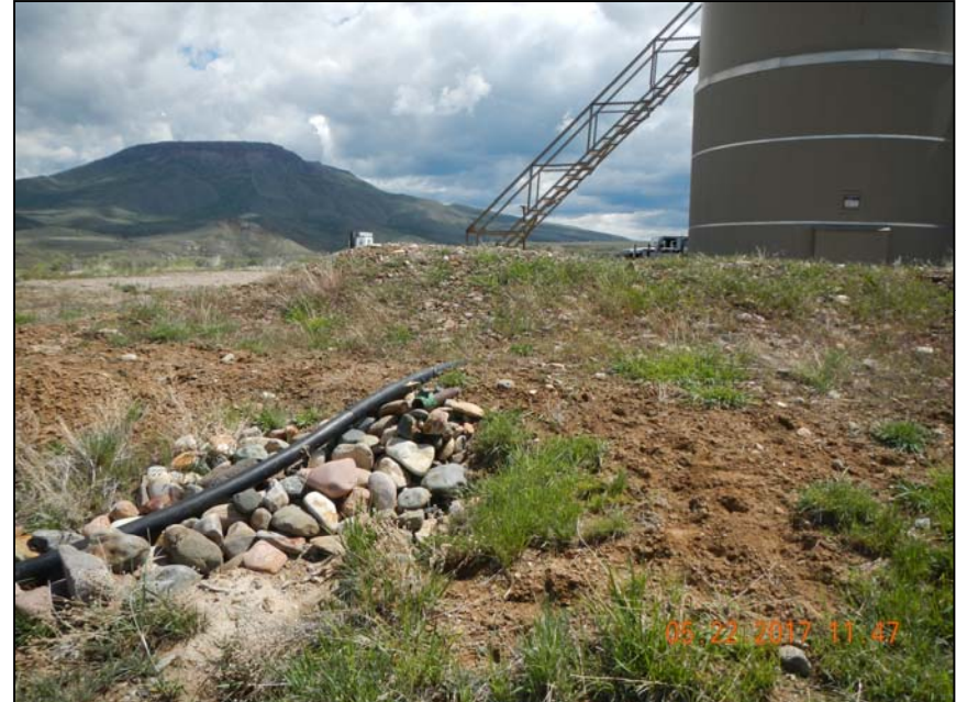
Photo 11. Poly and steel line from left photo. Poly line from tank. No point A identified for steel line.
