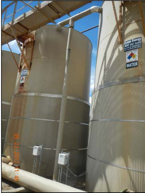
Photo 8. 2 -4" insulated flowlines going into 6" insulated line at base.
