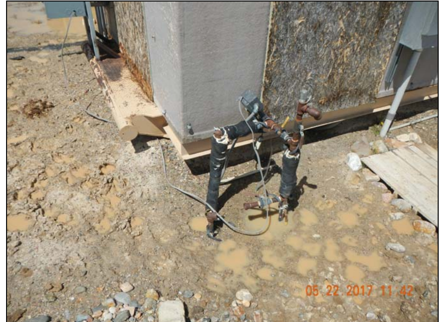
Photo 5. 2 -1” insulated risers at compressor corner.
