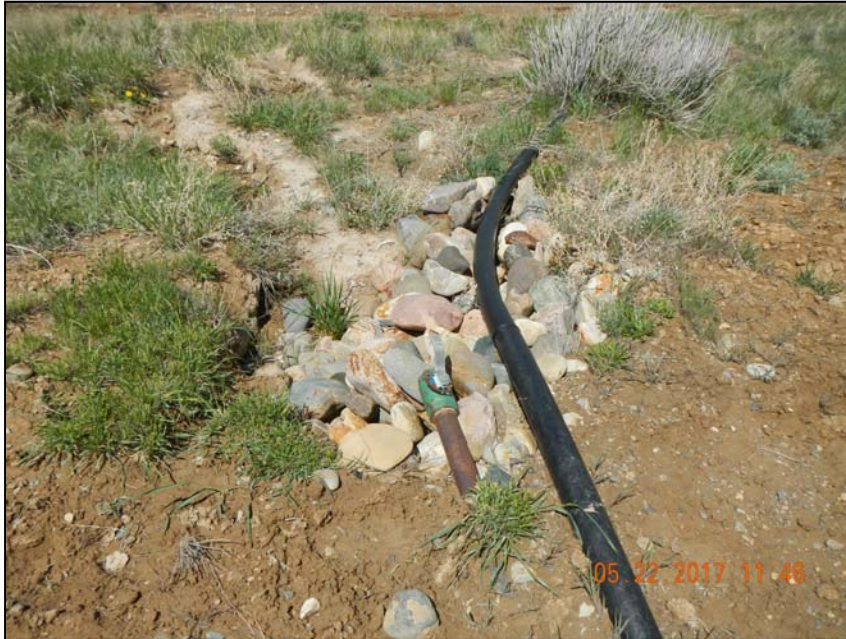
Photo 10. 1 -2" poly flowline. 1 -2" steel flowline.
