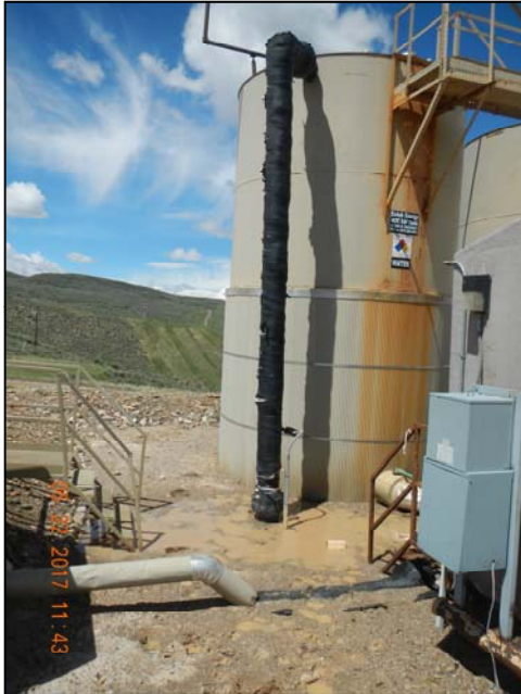
Photo 6. 1 -6" insulated flowline from tank. 1 - 4"insulated flowline from meter run.
