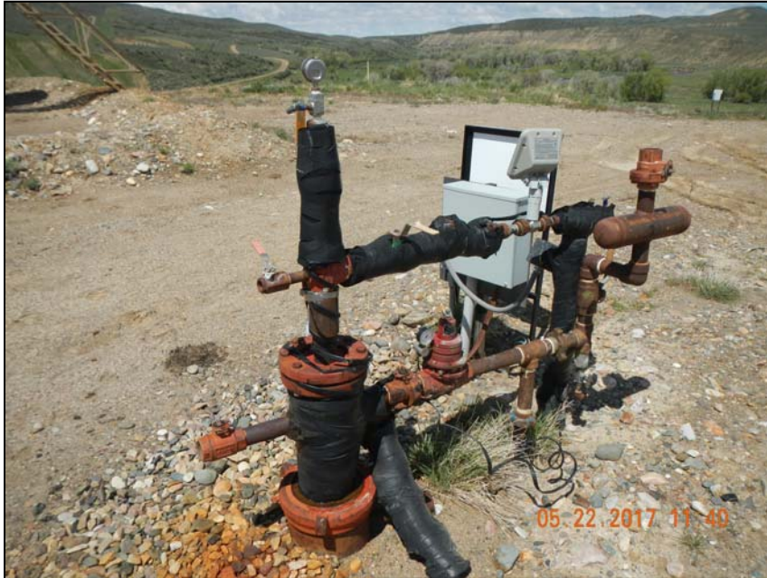
Photo 2. 1 -2" steel riser and 1 -2" insulated riser at wellhead.
