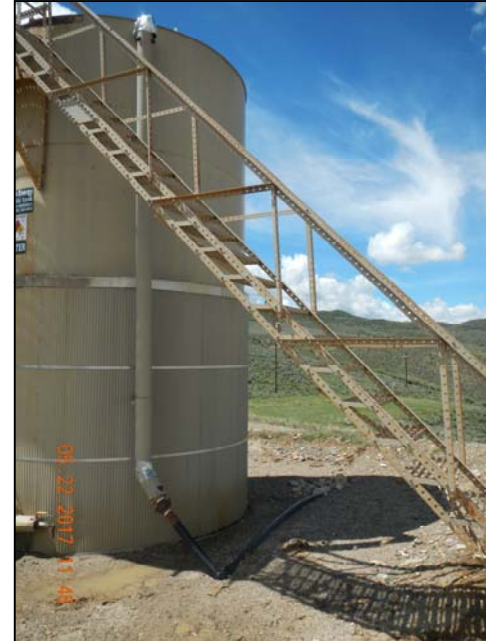
Photo 9. 1 -2" insulated flowline changing to poly line at tank base.
