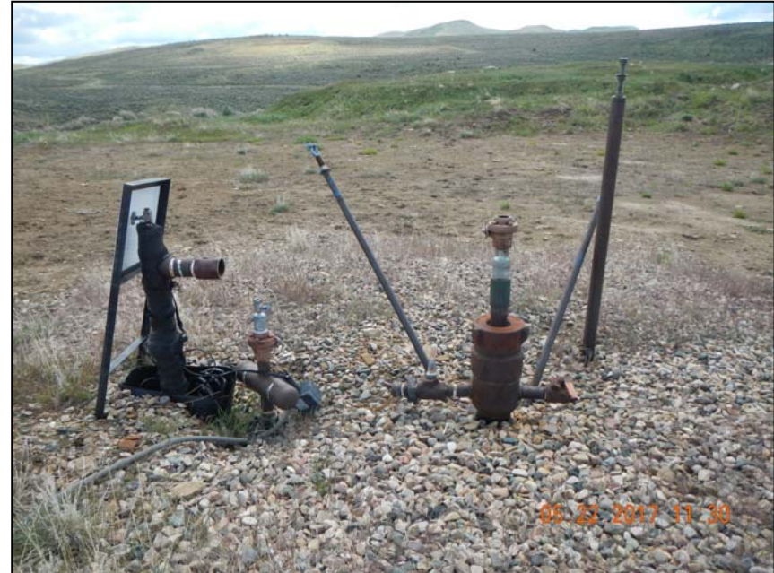
Photo 2. 2 -2" and 1 - 3" steel risers at wellhead
