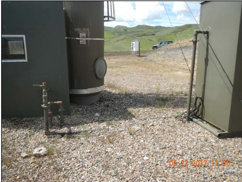
Photo 4. 2 -2" steel risers at separator and dehydrator.
