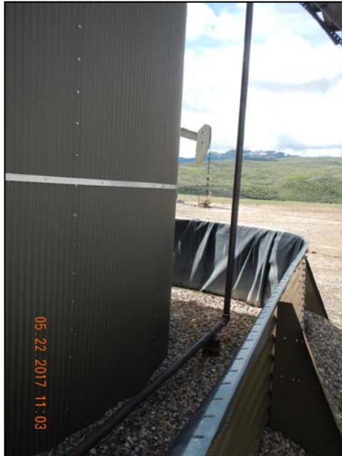
Photo 6. 1- 2" steel flowline from tank top.
