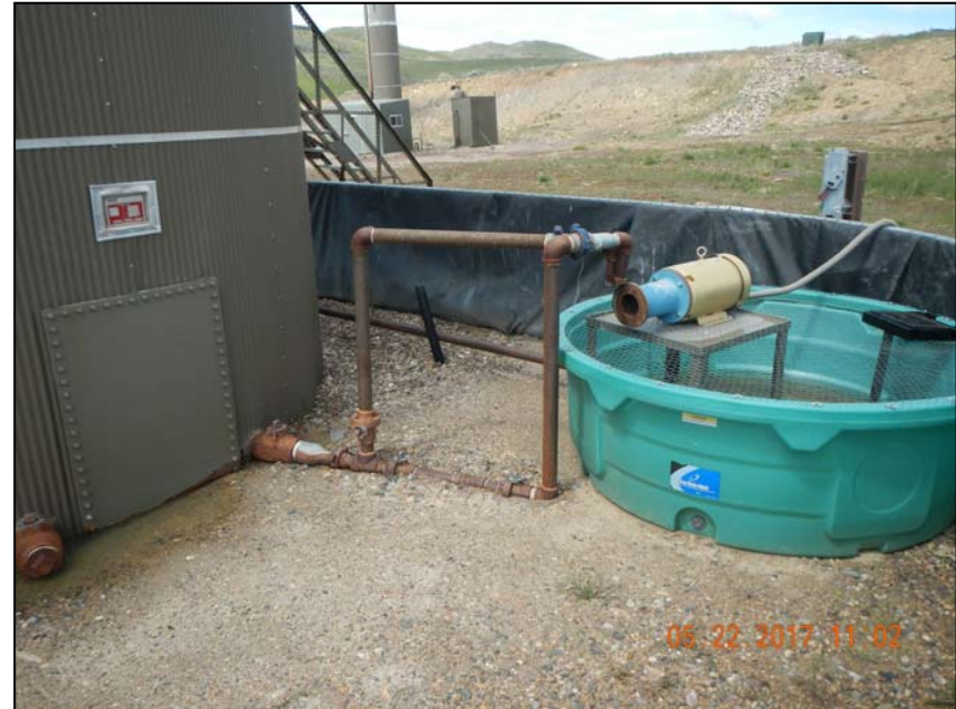
Photo 7. 2" line from left picture in background. 2 -2" steel risers from tank.
