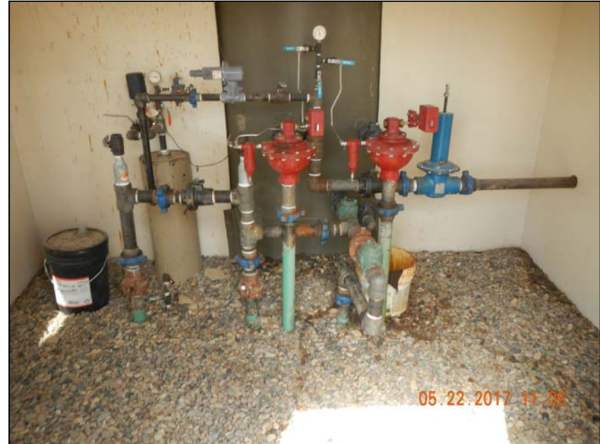
Photo 3. 5 - 2" steel risers inside separator shack
