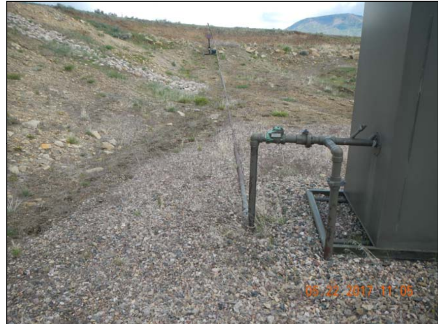
Photo 5. 1 -2" steel riser. 1 -2" steel flowline going to flare visible in background.
