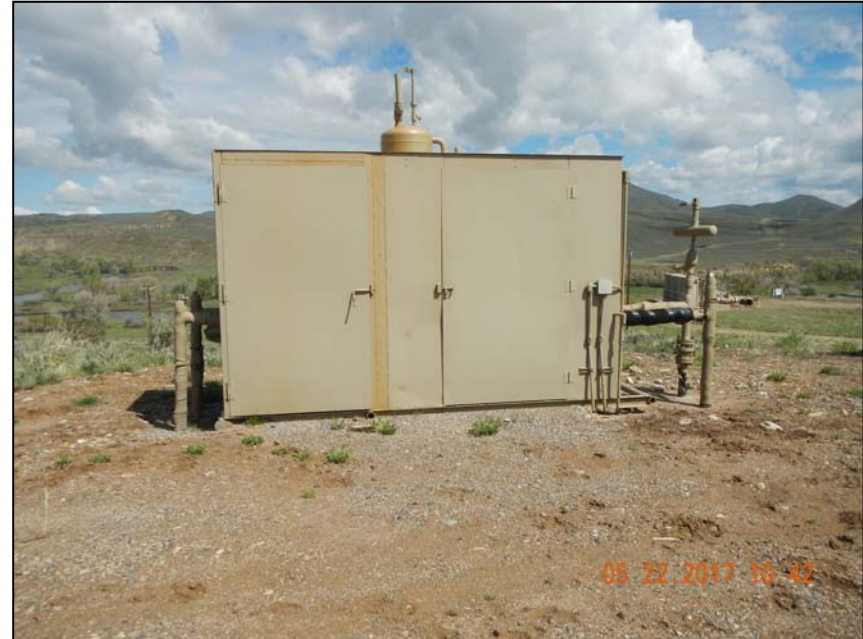
Photo 5. Dehydrator with 2 -2" risers on each side.
