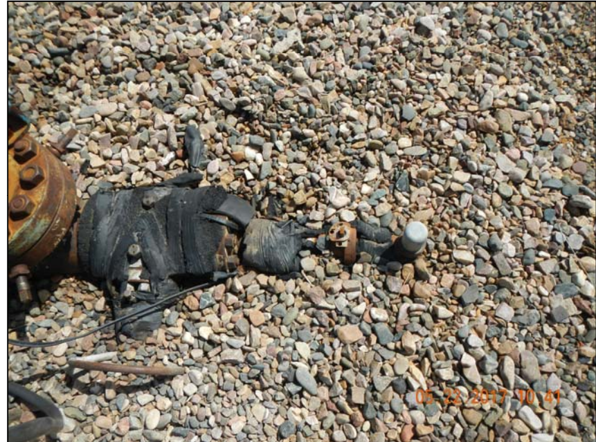
Photo 3. 1 -2" steel riser with no marking and no LOTO.
