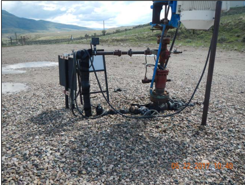
Photo 2. 2 -2" insulated risers at wellhead.
