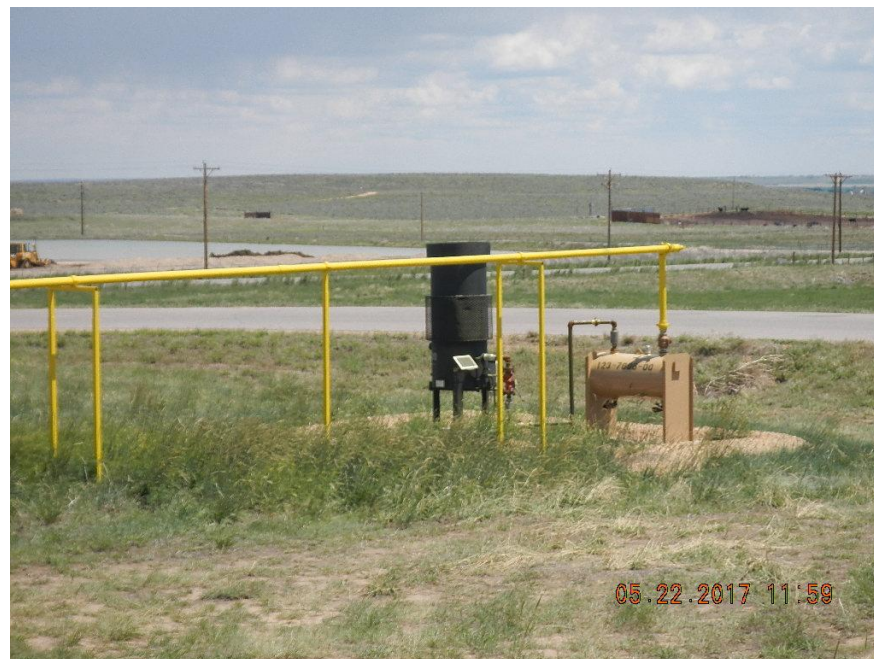
Emission Control Burner (new) from southwest.
