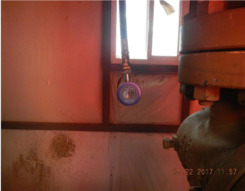
Digital gauge inside well shack, Reading: 1415 PSI
