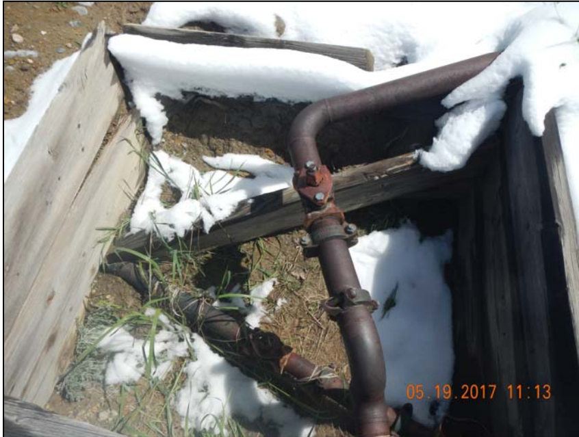
Photo 9. 3" and 4" steel risers at manifold between tank and separator.
