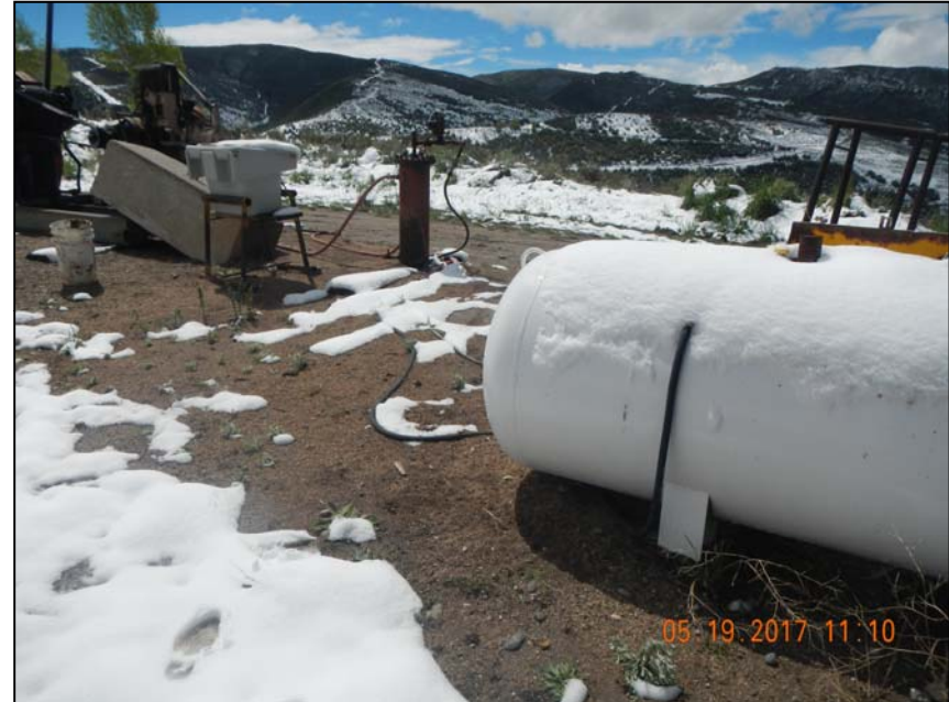
Photo 4. 2 - 1" poly lines extending from separator to propane tank and pump jack motor.
