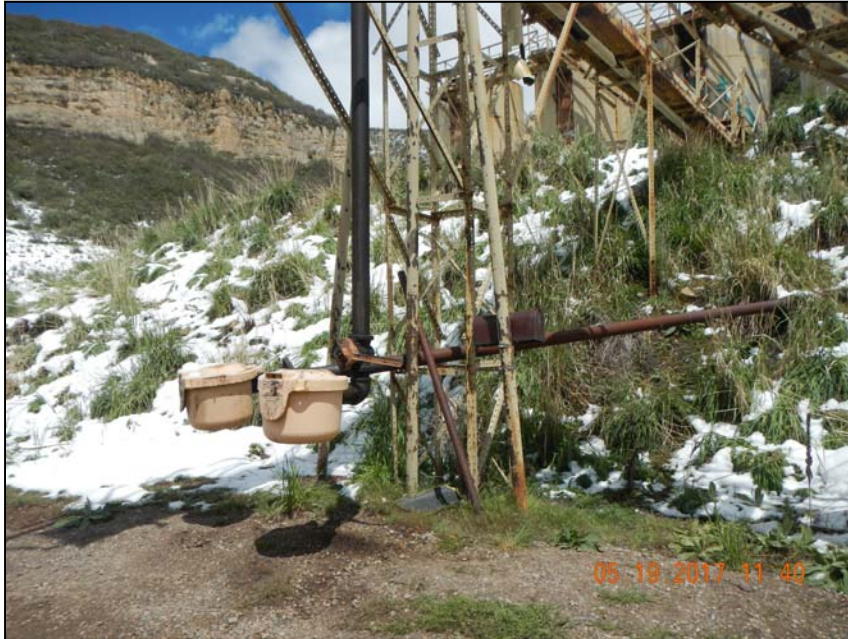
Photo 11. 2 – 4” steel flowlines at tank load out at base of hill.
