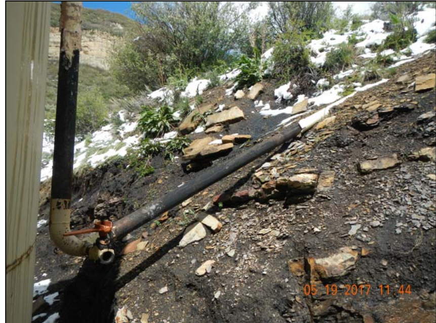
Photo 14. 4" steel flowline from uphill at wellhead.
