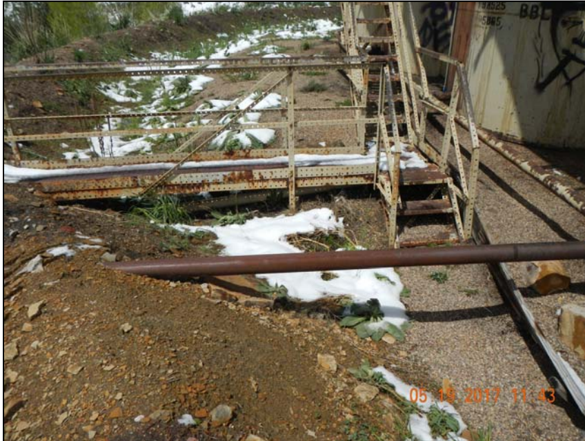
Photo 13. 2 – 4" steel flowlines at tanks.
