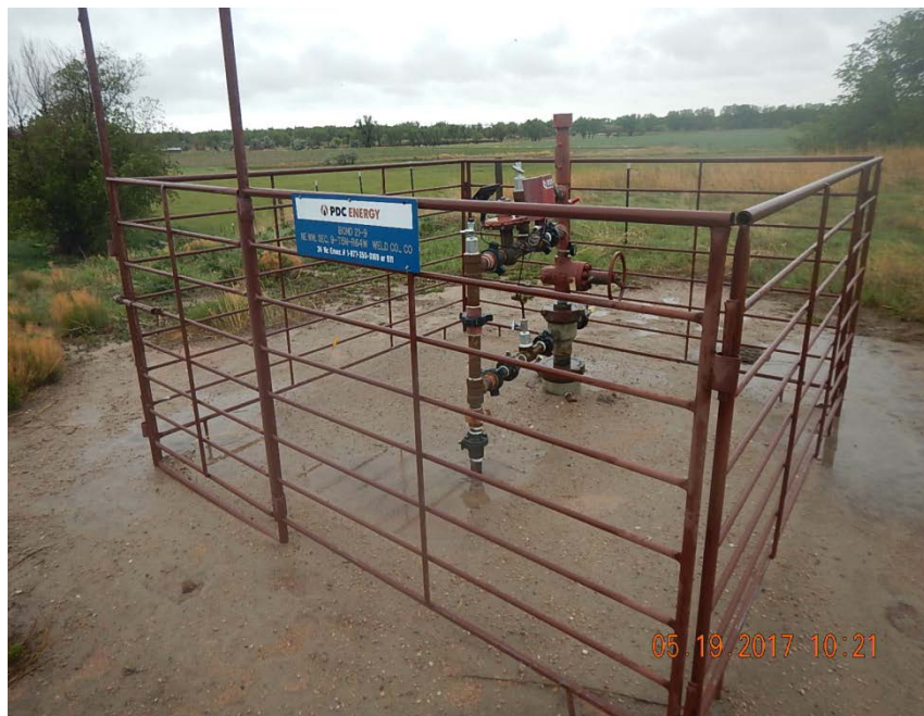
Photo 1: Flowlines at wellhead
