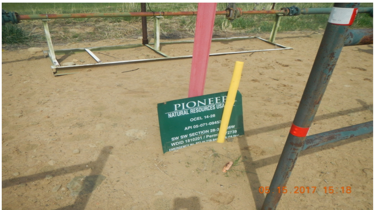
photo 4: Well sign is not appropriately attached.
