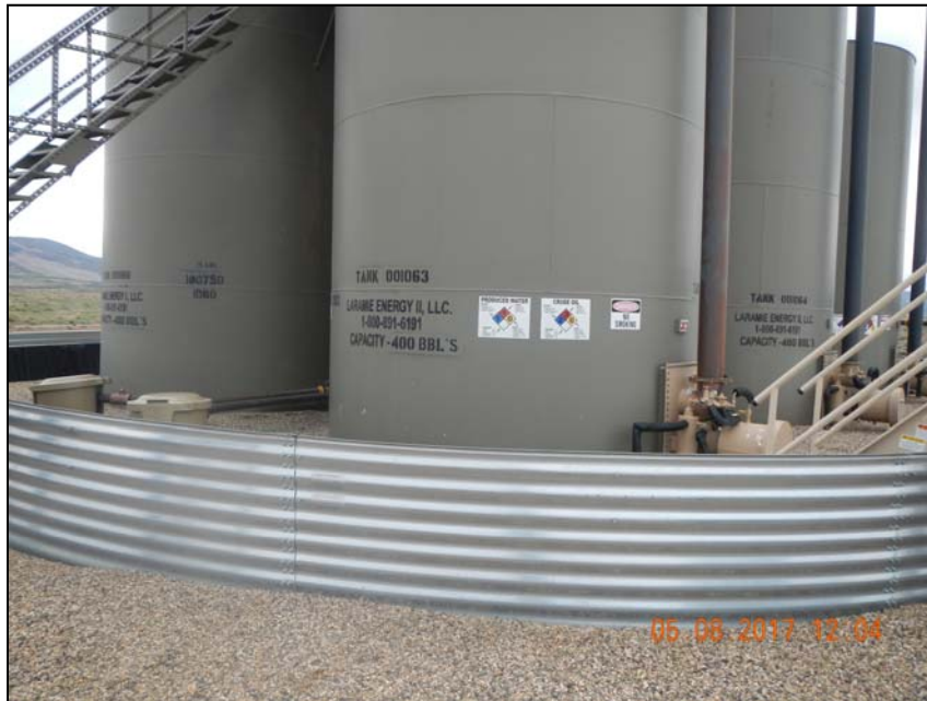
Photo 3. Tanks labeled with multiple contents.
