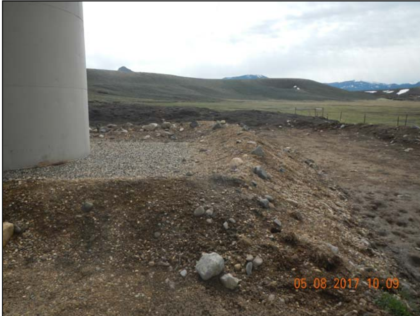
Photo 2. Unconsolidated, pervious berm in foreground. Unprotected topsoil pile in background.
