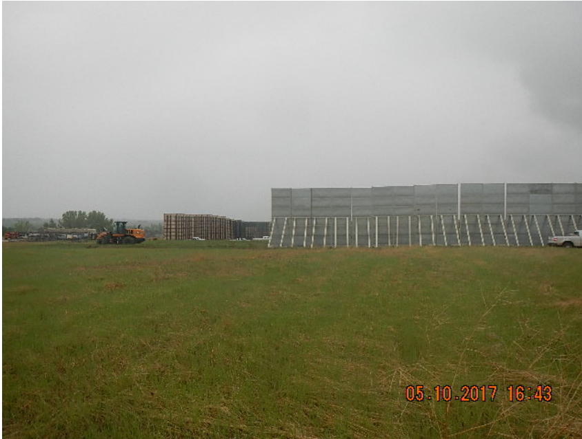
MOBLIE SOUND WALLS IN PROCESS OF BEING INSTALLED ON SOUTH END AND 32' SOUND WALLS ON WEST OF LOCATION
