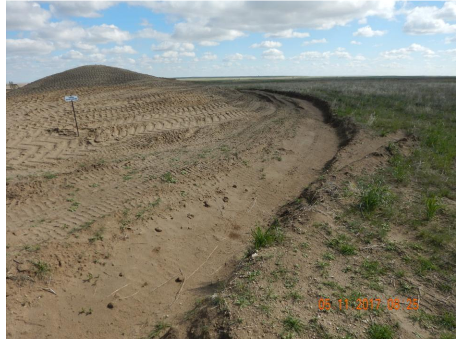
Photo 10: Photo taken from the southeast end of the location, facing north. Photo shows perimeter ditch remains constructed with a steep grade and/or have not been consolidated.
