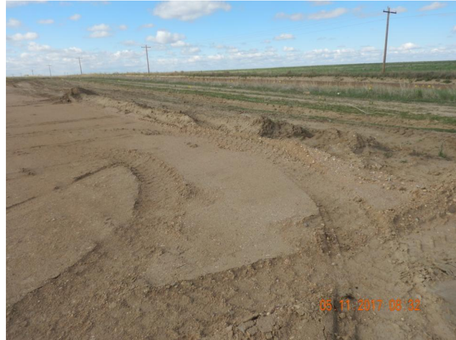
Photo 20: Photo taken from the northwest end of the location, facing southwest. Photo shows berms on the location have do not appear to be consolidated.
