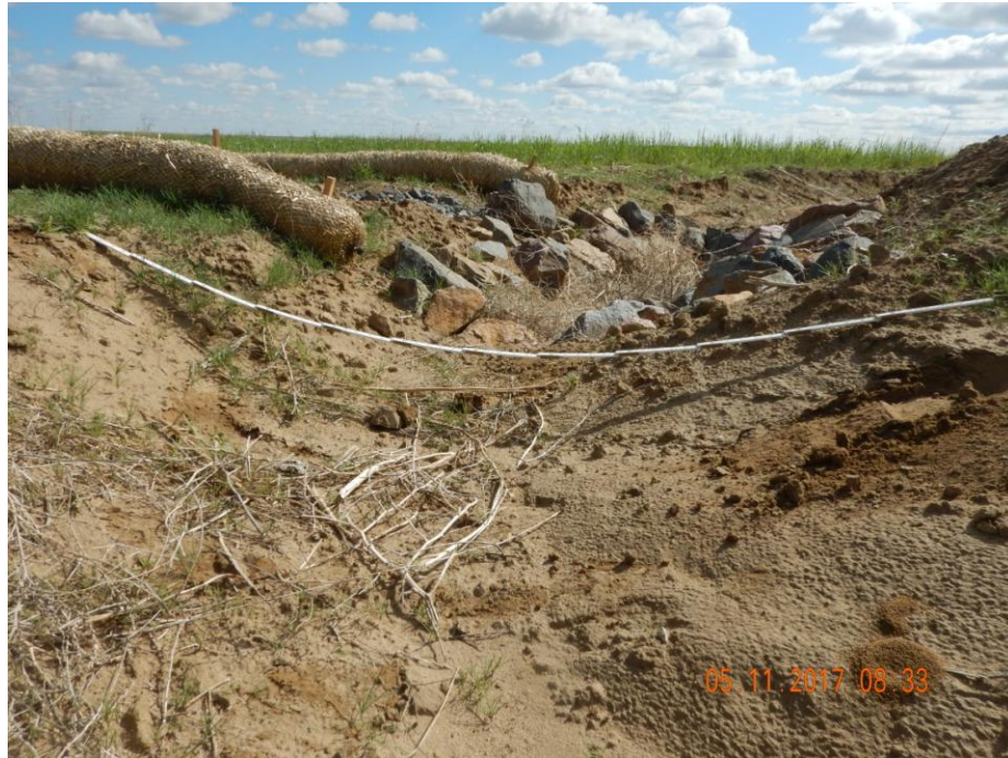
Photo 24: Photo taken from the sediment trap on the northwest end of the location. Per on-site conversations between BBC and COGCC staff 4/6/2017, sediment trap on location was determined to not have been constructed with good engineering practices. FIRR #401258682 states "Sediment traps were enlarged, smaller diameter aggregate placed at inlet and outlet. Outlet equipped with some type of filter media (straw wattle or hay bale)". Wattles have been installed; wattles are barriers that pond run off and do not filter stormwater. Wattles will not allow for adequate stormwater discharge from a sediment trap and should not be incorporated at the outlet of the sediment traps. Inlet armoring does not appear to be sufficient. 6 foot measuring stick for reference.
