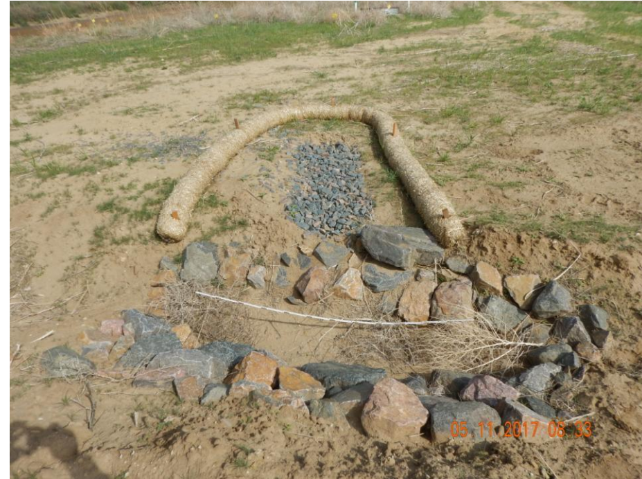
Photo 23: Photo taken from the sediment trap on the northwest end of the location. Per on-site conversations between BBC and COGCC staff 4/6/2017, sediment trap on location was determined to not have been constructed with good engineering practices. FIRR #401258682 states "Sediment traps were enlarged, smaller diameter aggregate placed at inlet and outlet. Outlet equipped with some type of filter media (straw wattle or hay bale)". Wattles have been installed; wattles are barriers that pond run off and do not filter stormwater. Wattles will not allow for adequate stormwater discharge from a sediment trap and should not be incorporated at the outlet of the sediment traps. Inlet armoring does not appear to be sufficient. 6 foot measuring stick for reference.
