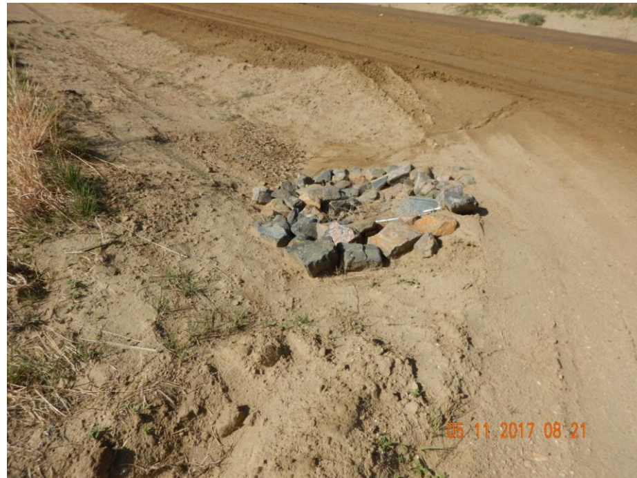
Photo 4: Photo taken from access road on the southwest end of the location. Photo shows culvert with rock armoring.
