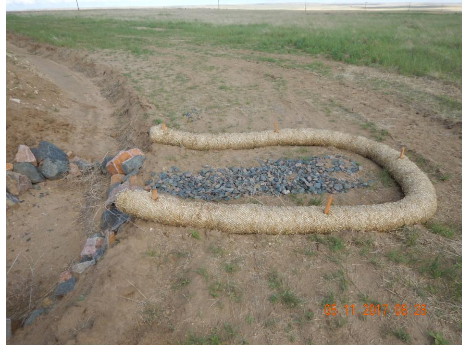
Photo 14: Photo taken from the sediment trap on the northeast end of the location. Per on-site conversations between BBC and COGCC staff 4/6/2017, sediment trap on location was determined to not have been constructed with good engineering practices. FIRR #401258682 states "Sediment traps were enlarged, smaller diameter aggregate placed at inlet and outlet. Outlet equipped with some type of filter media (straw wattle or hay bale)". Wattles have been installed; wattles are barriers that pond run off and do not filter stormwater. Wattles will not allow for adequate stormwater discharge from a sediment trap and should not be incorporated at the outlet of the sediment traps. Inlet armoring does not appear to be sufficient.
