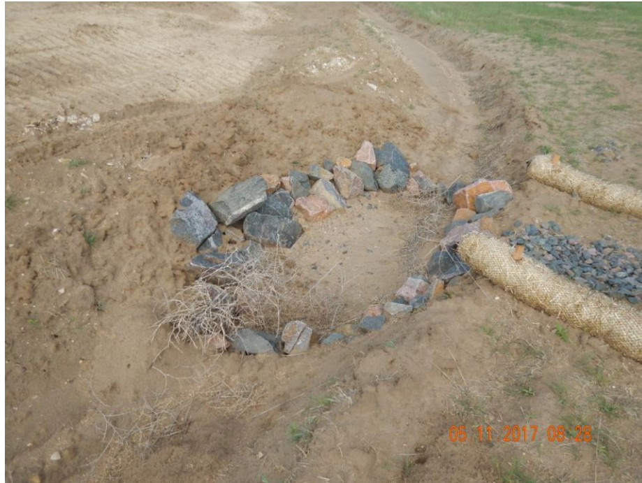
Photo 13: Photo taken from the sediment trap on the northeast end of the location. Per on-site conversations between BBC and COGCC staff 4/6/2017, sediment trap on location was determined to not have been constructed with good engineering practices. FIRR #401258682 states "Sediment traps were enlarged, smaller diameter aggregate placed at inlet and outlet. Outlet equipped with some type of filter media (straw wattle or hay bale)". Wattles have been installed; wattles are barriers that pond run off and do not filter stormwater. Wattles will not allow for adequate stormwater discharge from a sediment trap and should not be incorporated at the outlet of the sediment traps. Inlet armoring does not appear to be sufficient.
