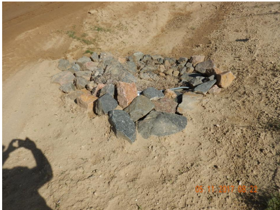
Photo 5: Photo taken from access road on the southwest end of the location. Photo shows culver with rock armoring.
