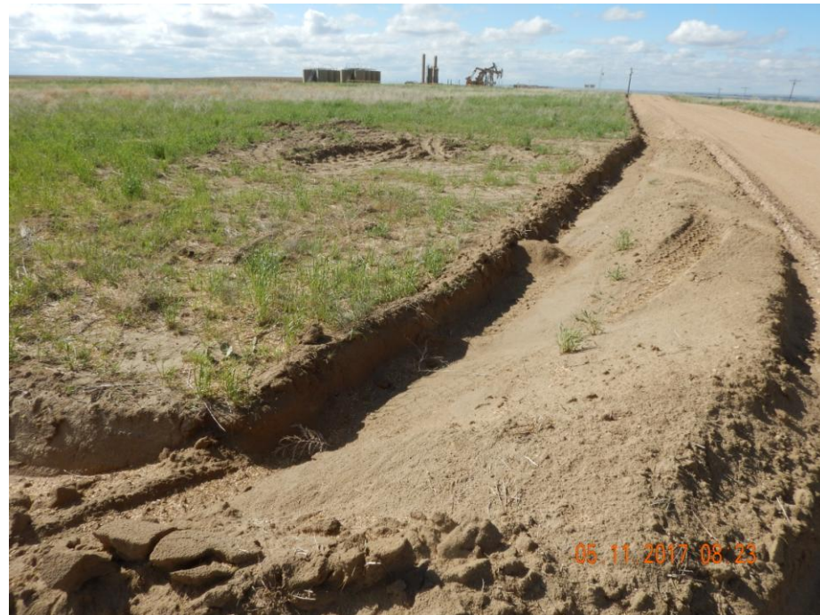
Photo 6: Photo taken from the southwest end of the location, facing south. Photo shows perimeter ditch remains constructed with a steep grade and/or have not been consolidated.
