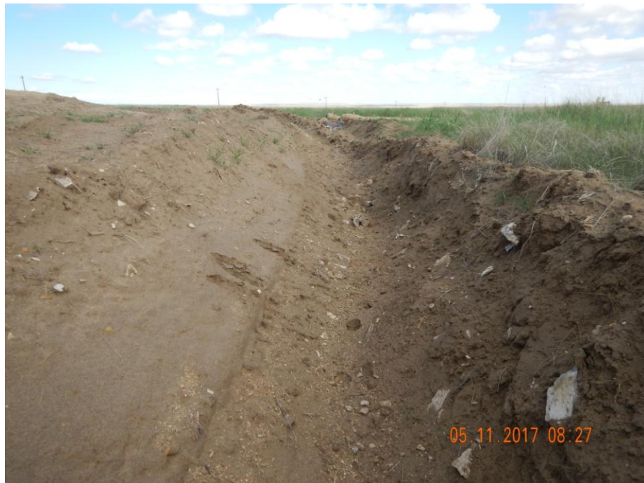
Photo 11: Photo taken from the southeast end of the location, facing north. Photo shows perimeter ditch remains constructed with a steep grade and/or have not been consolidated.
