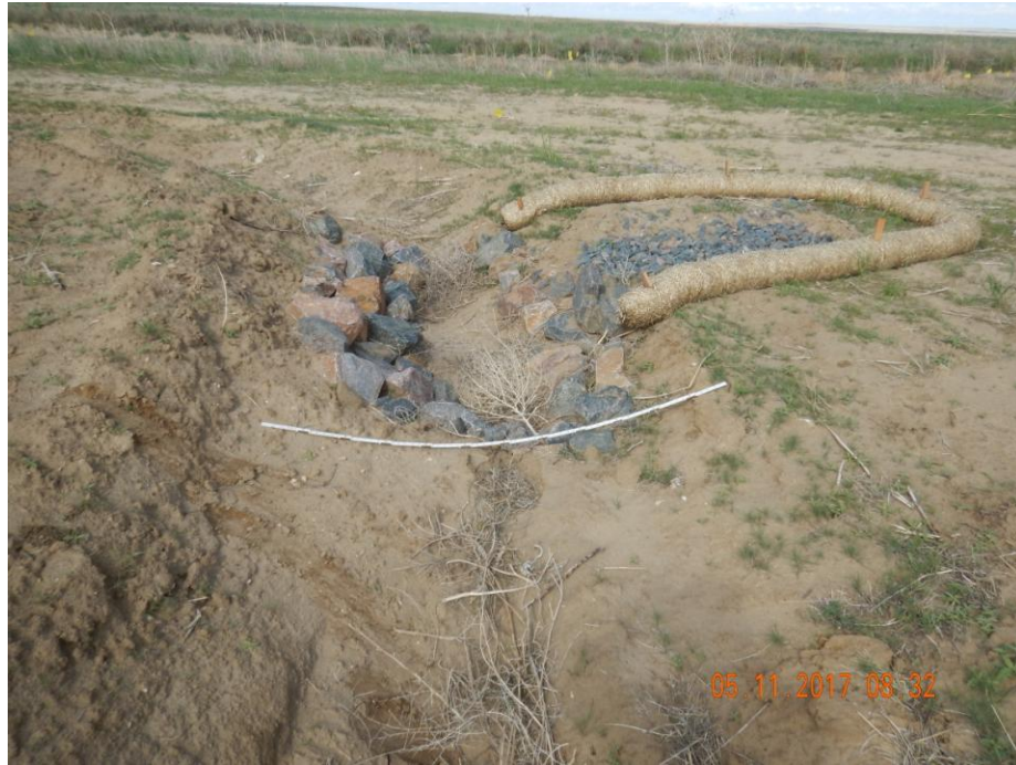
Photo 22: Photo taken from the sediment trap on the northwest end of the location. Per on-site conversations between BBC and COGCC staff 4/6/2017, sediment trap on location was determined to not have been constructed with good engineering practices. FIRR #401258682 states "Sediment traps were enlarged, smaller diameter aggregate placed at inlet and outlet. Outlet equipped with some type of filter media (straw wattle or hay bale)". Wattles have been installed; wattles are barriers that pond run off and do not filter stormwater. Wattles will not allow for adequate stormwater discharge from a sediment trap and should not be incorporated at the outlet of the sediment traps. Inlet armoring does not appear to be sufficient. 6 foot measuring stick for reference.
