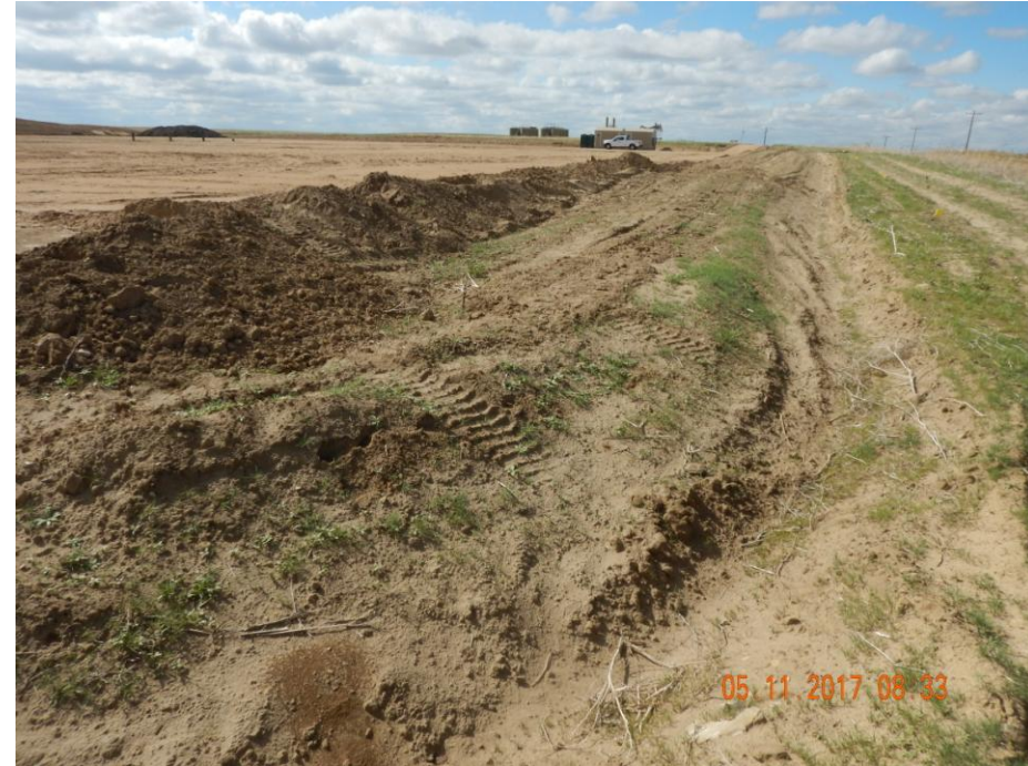
Photo 25: Photo taken from the northwest end of the location, facing south. Photo shows berms on the location have do not appear to be consolidated.
