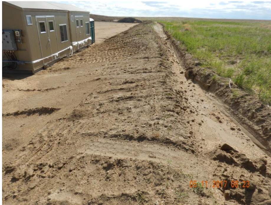
Photo 7: Photo taken from the southwest end of the location, facing east. Photo shows perimeter ditch remains constructed with a steep grade and/or have not been consolidated.
