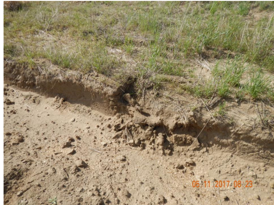
Photo 8: Photo taken from the south end of the location. Photo shows portions of the ditch that area beginning to “slough off”, or erode due to poor engineering along ditch.
