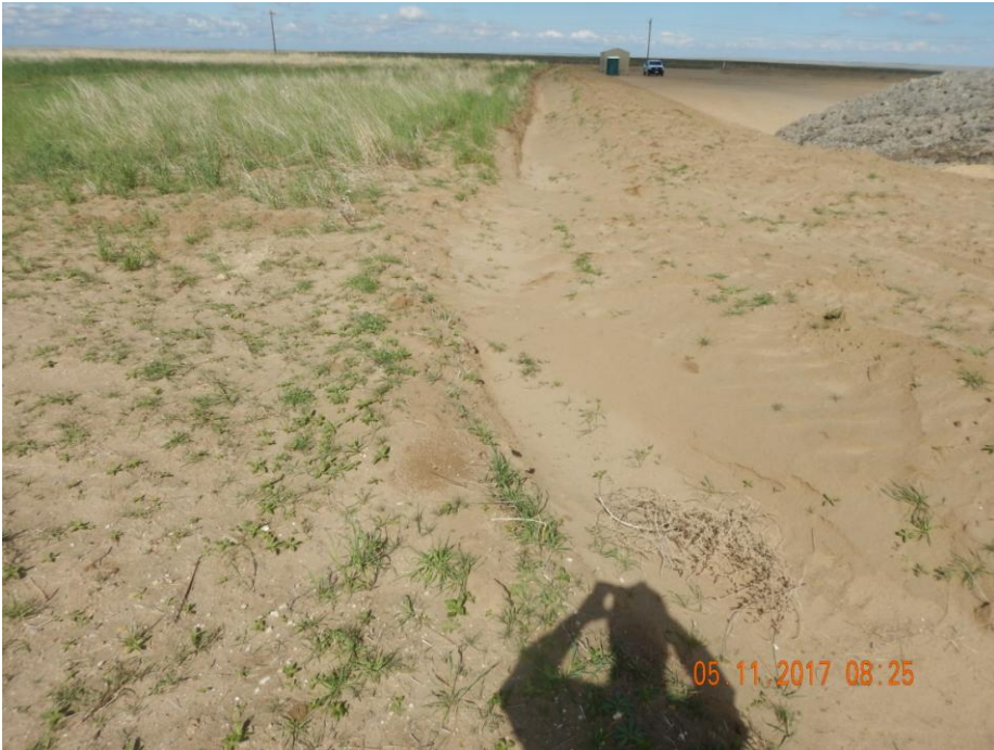
Photo 9: Photo taken from the southeast end of the location. Inspection #401245397 states “areas of the ditch has become filled w/ sediment and required maintenance”. FIRR #401258682 submitted by operator states “perimeter ditch maintenance conducted and sediment removed”. Photo shows ditch remains filled w/ sediment, maintenance has not been conducted as indicated by operator.
