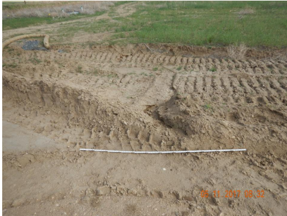
Photo 19: Photo taken from the northwest end of the location. Photo shows stormwater erosion has degraded the berm and slope of the location. Berms do not appear to be sufficiently consolidated on this area of the location. Vehicle traffic appears to have rendered the berm inadequate and allowed for stormwater degradation. 6 foot measuring stick for reference.
