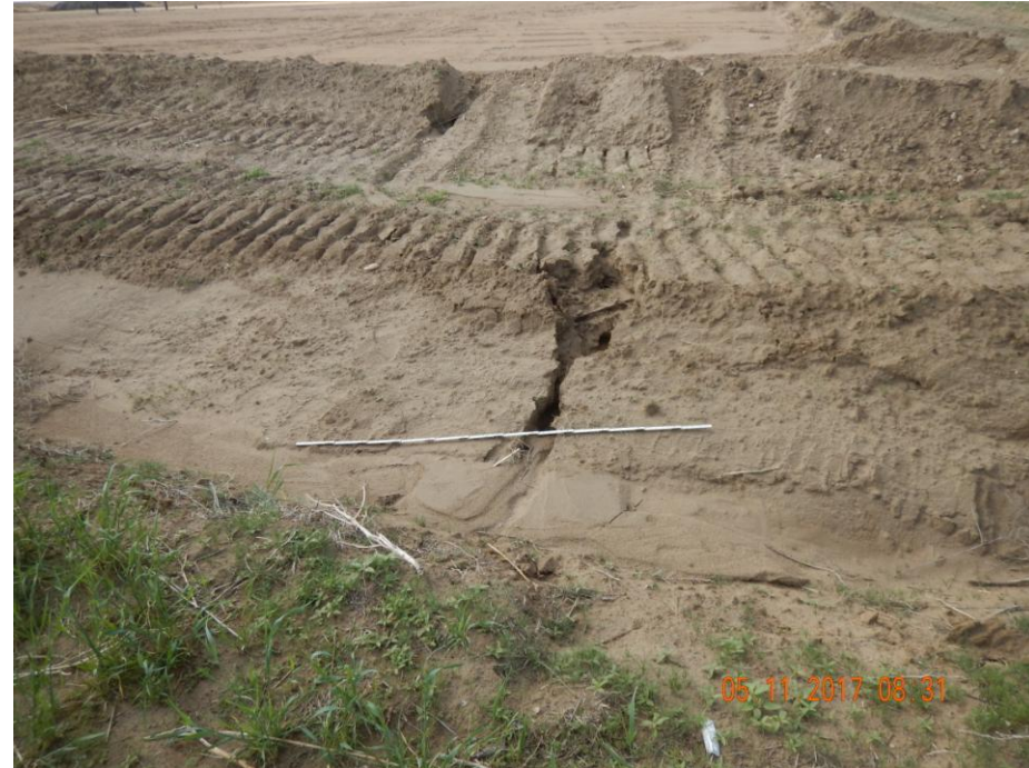
Photo 16: Photo taken from the northwest end of the location. Photo shows stormwater erosion has degraded the berm /slope/ditch of the location. Berms do not appear to be sufficiently consolidated on this area of the location. 6 foot measuring stick for reference.
