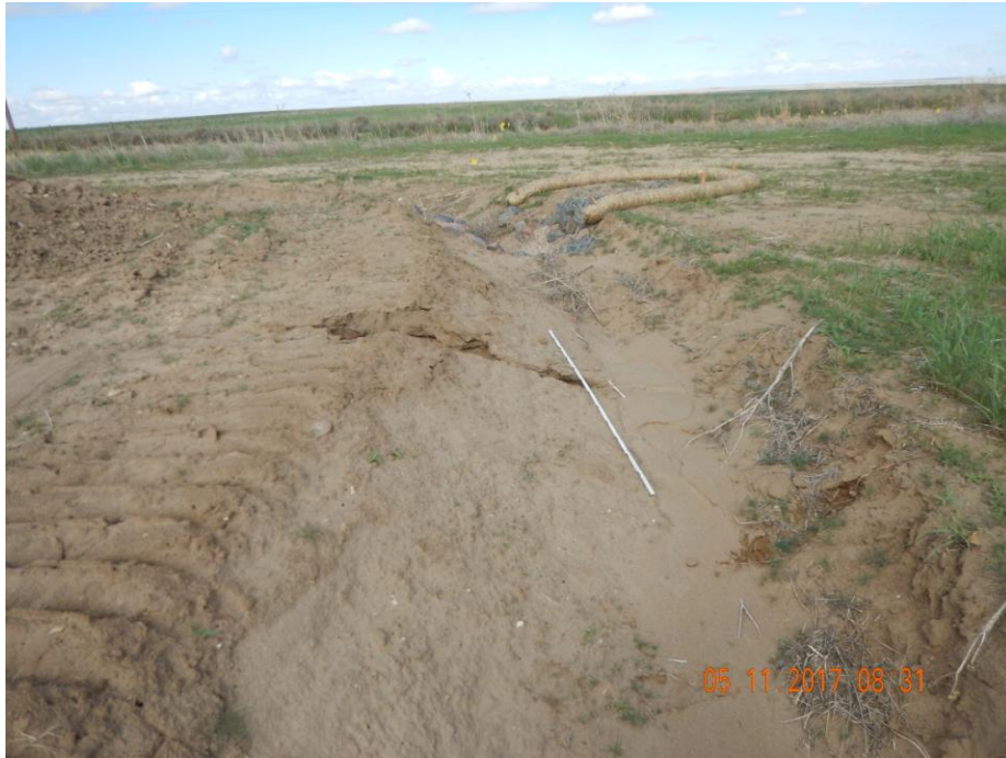
Photo 17: Photo taken from the northwest end of the location. Photo shows stormwater erosion has degraded the berm/slope/ditch of the location. Berms do not appear to be sufficiently consolidated on this area of the location. 6 foot measuring stick for reference.
