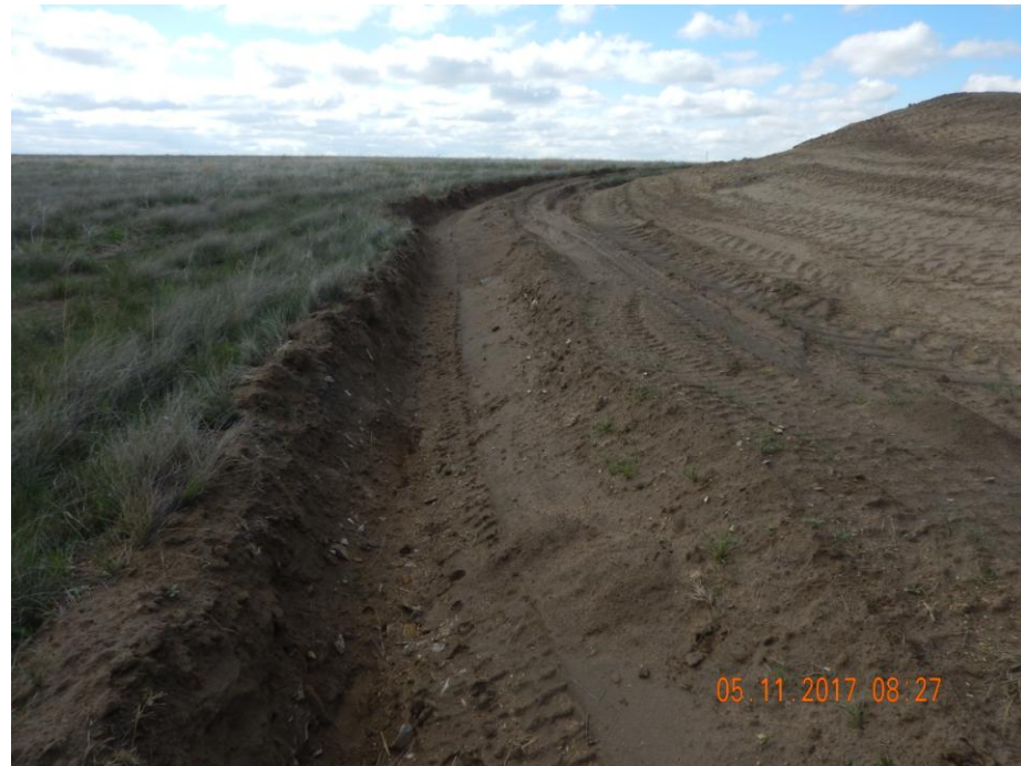
Photo 12: Photo taken from the northeast end of the location, facing south. Photo shows perimeter ditch remains constructed with a steep grade and/or have not been consolidated.
