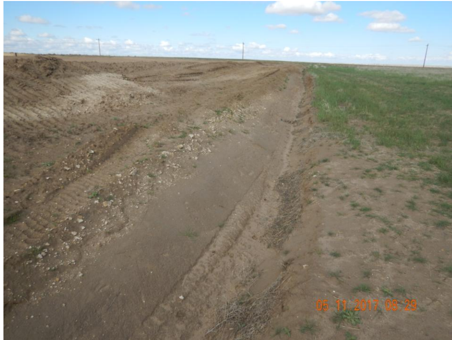
Photo 15: Photo taken from the northeast end of the location, facing west. Photo shows perimeter ditch remains constructed with a steep grade and/or have not been consolidated.
