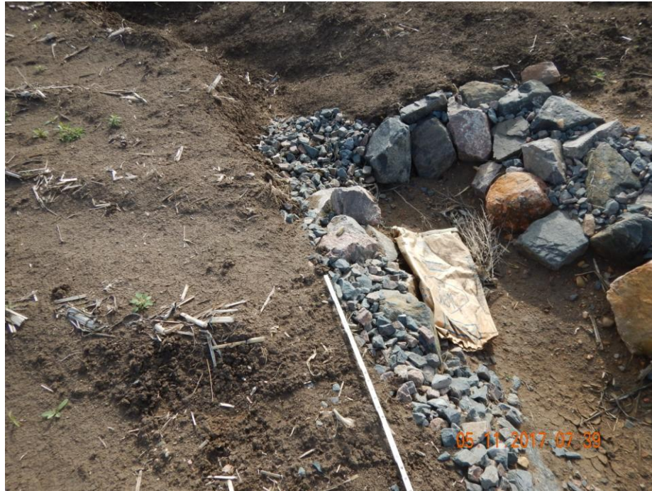
Photo 7: Photo taken from the sediment trap on the northwest end of the location. FIRR #401258606 states "Sediment traps were enlarged, smaller diameter aggregate placed at inlet and outlet. Outlet equipped with some type of filter media (straw wattle or hay bale)". This is the only trap for the entire location. Per on-site conversations between BBC and COGCC staff, sediment trap on location was determined to not have been constructed with good engineering practices. No improvements have been made since these discussions; trap has not been enlarged w/ filter media. Inlet armoring does not appear to be sufficient.
