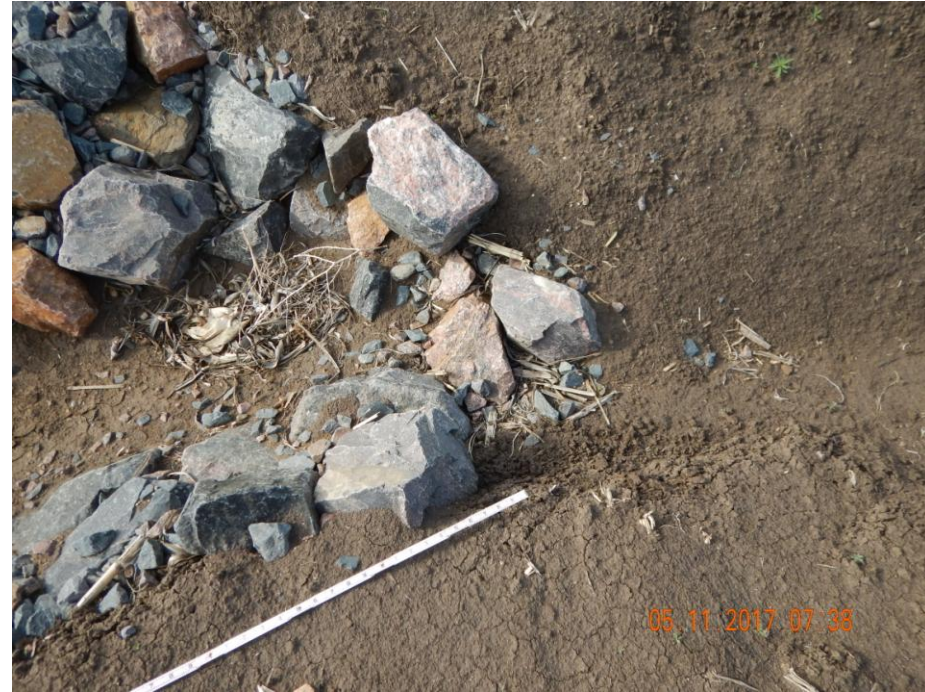
Photo 6: Photo taken from the sediment trap on the northwest end of the location. FIRR #401258606 states "Sediment traps were enlarged, smaller diameter aggregate placed at inlet and outlet. Outlet equipped with some type of filter media (straw wattle or hay bale)". This is the only trap for the entire location. Per on-site conversations between BBC and COGCC staff, sediment trap on location was determined to not have been constructed with good engineering practices. No improvements have been made since these discussions; trap has not been enlarged w/ filter media. Inlet armoring does not appear to be sufficient.
