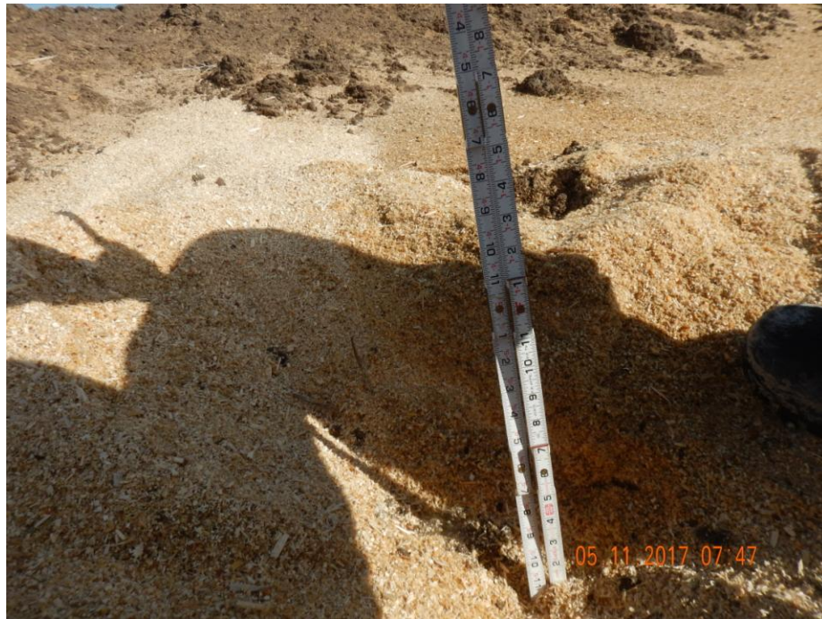
Photo 22: Photo taken from the southeast end of the location. Photo shows what appears to be saw dust has blown from the location and begun inundating the ditch. Saw dust has filled the ditch up over a foot in some areas. Advise removing before ditch is no longer in proper functioning condition.
