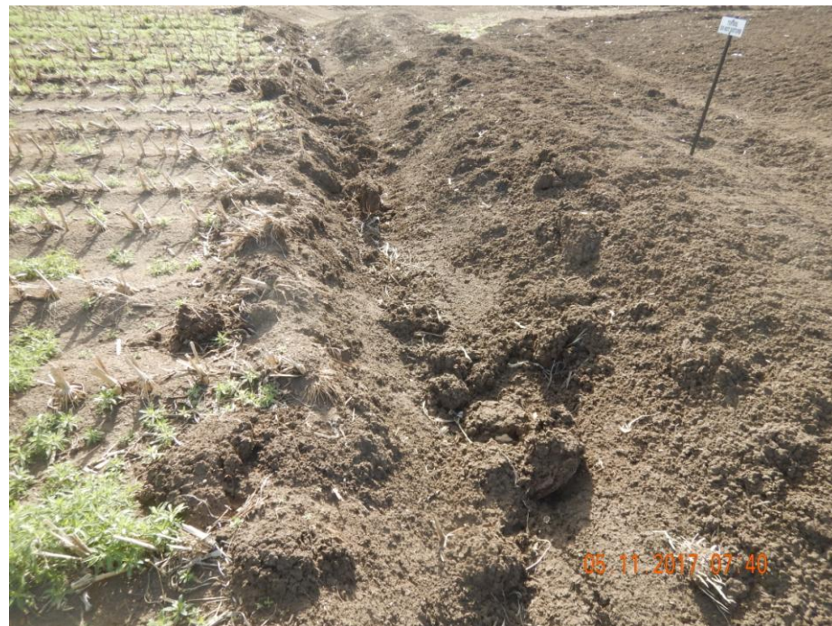
Photo 12: Photo taken from the ditch on the northeast end of the location. Photo shows ditch remain constructed with a steep grade and/or have not been consolidated. Soil has “sloughed off” from the walls in areas of the ditch.
