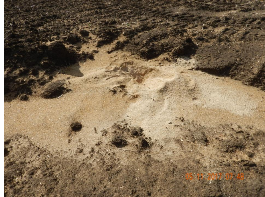
Photo 25: Photo taken from the southeast end of the location. Photo shows what appears to be saw dust has blown from the location and begun inundating the ditch. Saw dust has filled the ditch up over a foot in some areas. Advise removing before ditch is no longer in proper functioning condition.
