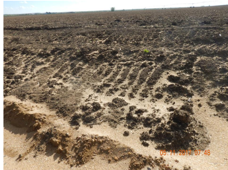
Photo 23: Photo taken from the southeast end of the location, facing east. FIRR #401258606 from operator states "The slopes on the eastern perimeter have been retracted". Photo shows that the slopes on the eastern perimeter of the location have not been retracted as stated in the FIRR.
