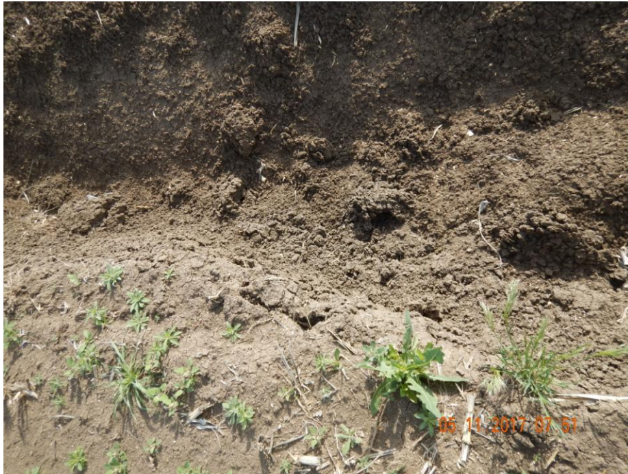
Photo 30: Photo taken from the ditch on the southwest end of the location. Photo shows ditch remain constructed with a steep grade and/or have not been consolidated. Photo also shows soil has “sloughed off” from the walls in areas of the ditch, or is beginning to erode off into the ditch.
