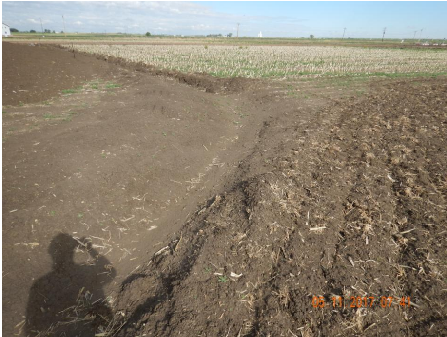
Photo 15: Photo taken from the northeast end of the location, facing north. Photo shows a low point in the northeast end; Per on-site conversations with BBC on 4/6/2017, COGCC staff were under the impression that additional BMPs to allow for adequate sediment laden free stormwater discharge would be installed on the northeast end of the location.
