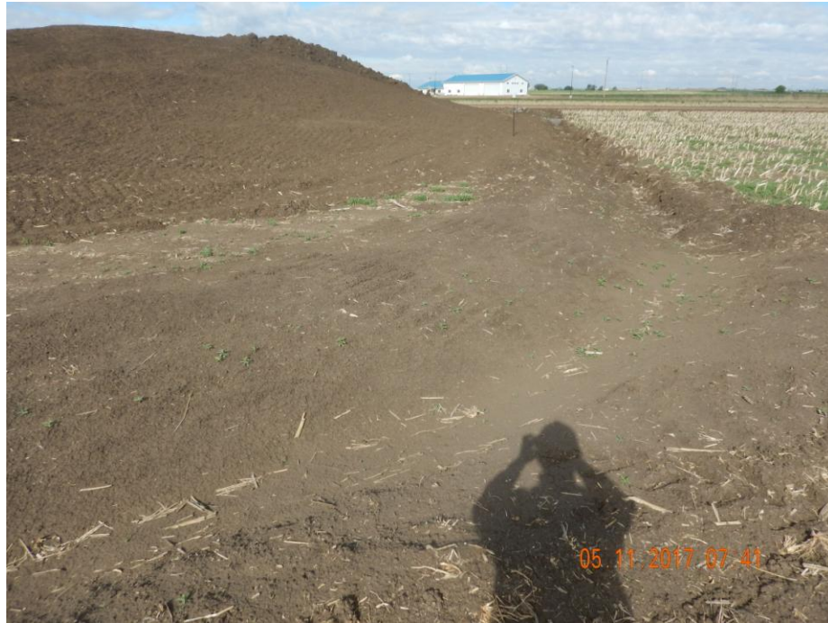
Photo 13: Photo taken from the northeast end of the location, facing west. Photo shows a low point in the northeast end; Per on-site conversations with BBC on 4/6/2017, COGCC staff were under the impression that additional BMPs to allow for adequate sediment laden free stormwater discharge would be installed on the northeast end of the location.
