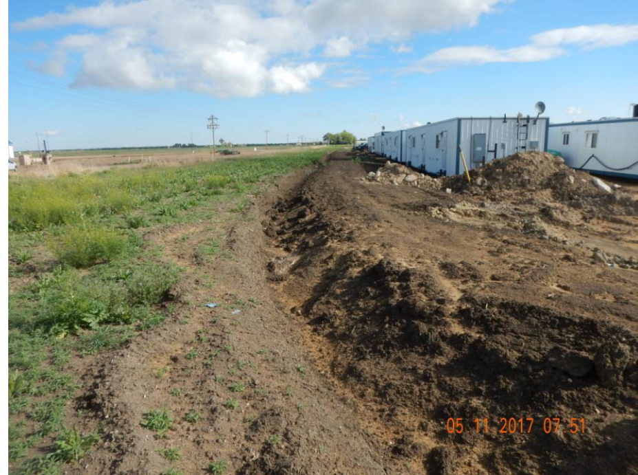
Photo 29: Photo taken from the ditch on the southwest end of the location, facing north. Photo shows ditch remains constructed with a steep grade and/or have not been consolidated. Photo also shows soil has “sloughed off” from the walls in areas of the ditch, or is beginning to erode off into the ditch.
