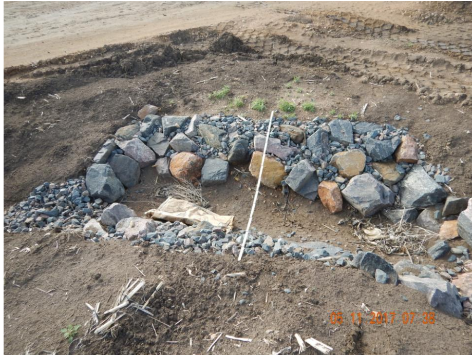
Photo 5: Photo taken from the sediment trap on the northwest end of the location. FIRR #401258606 states "Sediment traps were enlarged, smaller diameter aggregate placed at inlet and outlet. Outlet equipped with some type of filter media (straw wattle or hay bale)". This is the only trap for the entire location. Per on-site conversations between BBC and COGCC staff, sediment trap on location was determined to not have been constructed with good engineering practices. No improvements have been made since these discussions; trap has not been enlarged w/ filter media. Inlet armoring does not appear to be sufficient. 6 foot measuring stick for reference.
