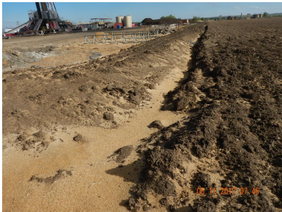
Photo 19: Photo taken from the southeast end of the location, facing north. Photo shows what appears to be saw dust has blown from the location and begun inundating the ditch.
