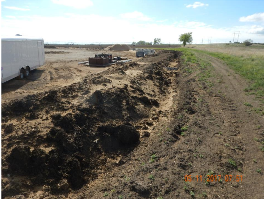
Photo 28: Photo taken from the ditch on the southwest end of the location, facing east. Photo shows ditch remains constructed with a steep grade and/or have not been consolidated. Photo also shows soil has “sloughed off” from the walls in areas of the ditch, or is beginning to erode off into the ditch.
