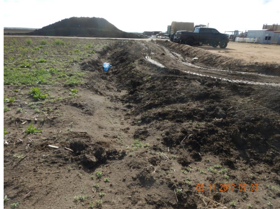
Photo 2: Photo taken from the northwest end of the location, facing east. Photo shows ditch along perimeter of the location. Ditches along perimeter location have been constructed with a step grade and/or have not been consolidated. Without proper consolidation and grade, ditch will increase the sediment laden stormwater runoff from the location.
