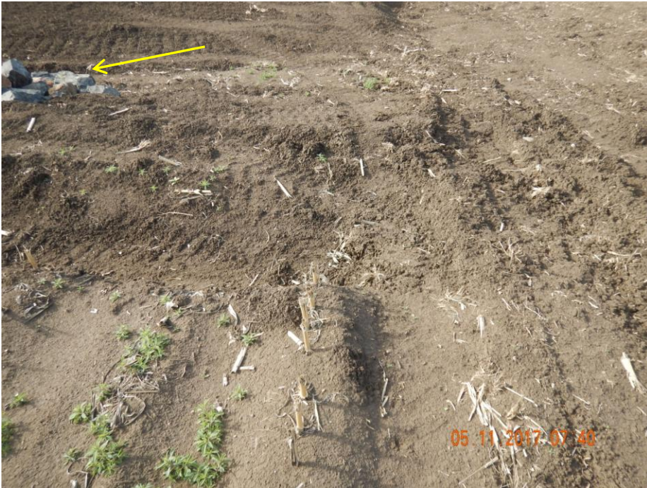
Photo 9: Photo taken from the northeast end of the location. Photo shows sediment trap that had previously existed has been removed (yellow arrow). Ditch on this portion of the location ends abruptly without any outlet BMP in place to allow for adequate sediment laden free stormwater discharge. Per on-site conversations with BBC on 4/6/2017, COGCC staff were under the impression that additional BMPs to allow for adequate sediment laden free stormwater discharge would be installed on the northeast end of the location.
