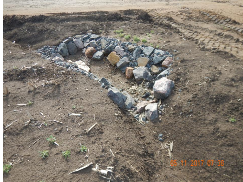
Photo 4: Photo taken from the sediment trap on the northwest end of the location. FIRR #401258606 states "Sediment traps were enlarged, smaller diameter aggregate placed at inlet and outlet. Outlet equipped with some type of filter media (straw wattle or hay bale)". This is the only trap for the entire location. Per on-site conversations between BBC and COGCC staff, sediment trap on location was determined to not have been constructed with good engineering practices. No improvements have been made since these discussions; trap has not been enlarged w/ filter media. Inlet armoring does not appear to be sufficient.
