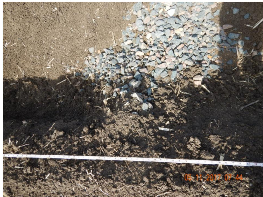
Photo 18: Photo taken from the ditch on the east end of the location. Photo also shows soil has “sloughed off” from the walls in areas of the ditch, or is beginning to erode off into the ditch. Rock aggregate is a check dam that has become inundated with sediment from the wall. 6 foot measuring stick for reference.
