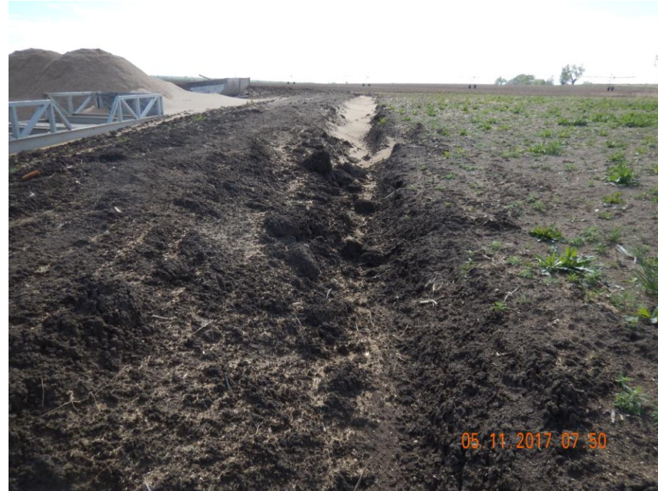
Photo 27: Photo taken from the ditch on the southwest end of the location, facing east. Photo shows ditch remains constructed with a steep grade and/or have not been consolidated. Photo also shows soil has “sloughed off” from the walls in areas of the ditch, or is beginning to erode off into the ditch.
