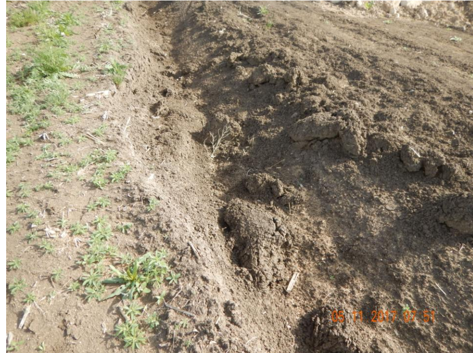
Photo 31: Photo taken from the ditch on the southwest end of the location. Photo shows ditch remain constructed with a steep grade and/or have not been consolidated. Photo also shows soil has “sloughed off” from the walls in areas of the ditch, or is beginning to erode off into the ditch.
