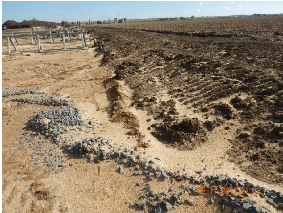
Photo 24: Photo taken from the southeast end of the location, facing north. FIRR #401258606 from operator states "The slopes on the eastern perimeter have been retracked". Photo shows that the slopes on the eastern perimeter of the location have not been retracked as stated in the FIRR.
