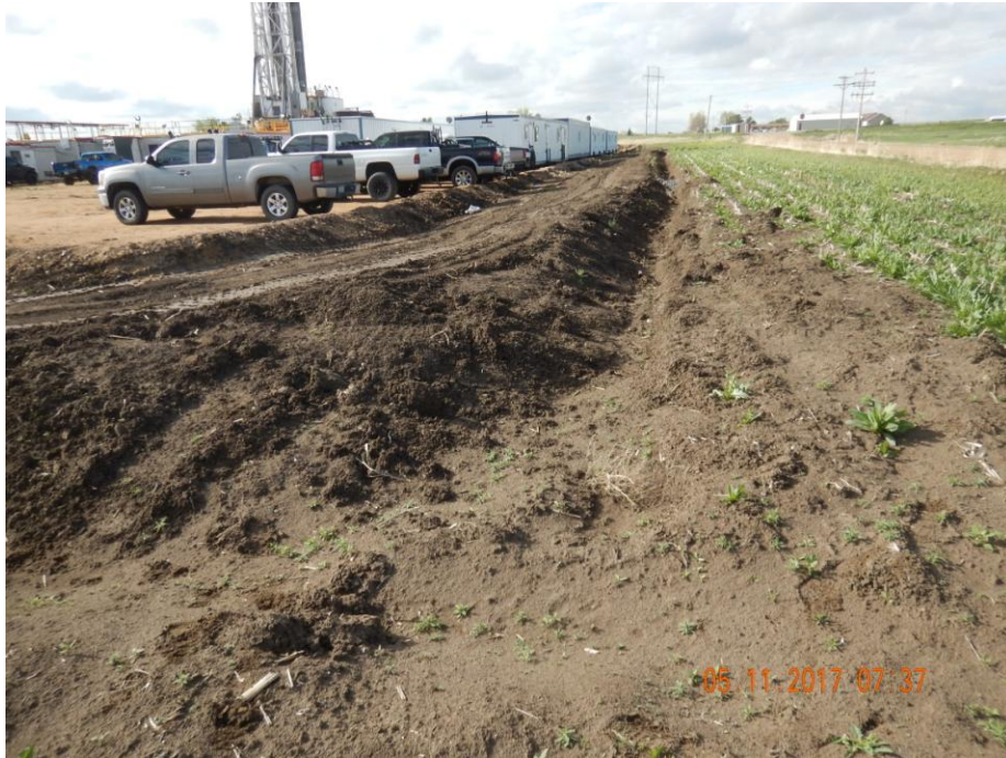
Photo 1: Photo taken from the northwest end of the location, facing south. Photo shows ditch along perimeter of the location. Ditches along perimeter location have been constructed with a step grade and/or have not been consolidated. Without proper consolidation and grade, ditch will increase the sediment laden stormwater runoff from the location.
