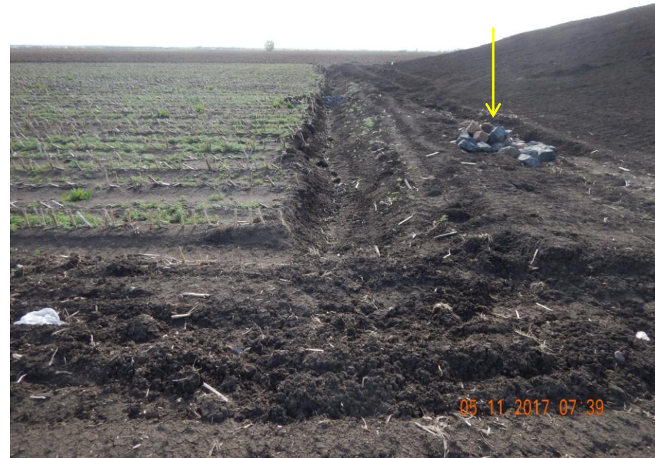
Photo 8: Photo taken from the northeast end of the location, facing east. Photo shows sediment trap that had previously existed has been removed (yellow arrow). Ditch on this portion of the location ends abruptly without any outlet BMP in place to allow for adequate sediment laden free stormwater discharge. Per on-site conversations with BBC on 4/6/2017, COGCC staff were under the impression that additional BMPs to allow for adequate sediment laden free stormwater discharge would be installed on the northeast end of the location.
