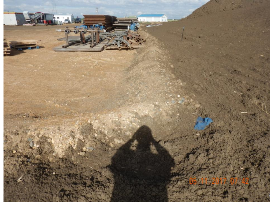
Photo 16: Photo taken from the north end of the location. Photo shows berms on location appear to be consolidated and in proper functioning condition.
