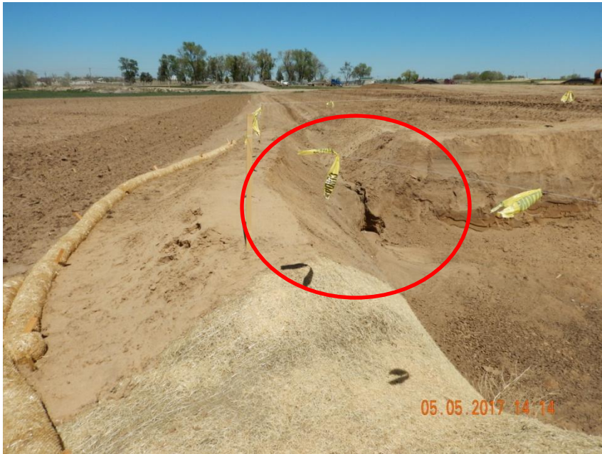
Photo 3. Photo taken from the sediment trap, facing East. Erosion is occurring at the inlet of the sediment trap because there is no inlet protection. May need to install inlet protection and monitor to ensure erosion does not progress further.
