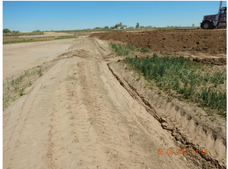
Photo 4. Photo taken from the northern location, facing East. A ditch and berm BMP has been installed around the perimeter of the location.
