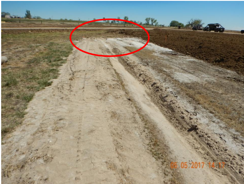
Photo 5. Photo taken from the northeastern location, facing Southeast. A ditch and berm BMP has been installed around the perimeter of the location but stops short along the northeastern location.
