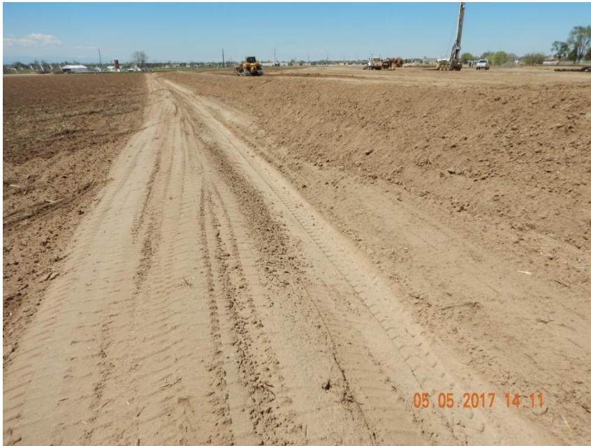
Photo 1. Photo taken from the southwestern location, facing North. A ditch and berm BMP has been installed around the perimeter of the location.
