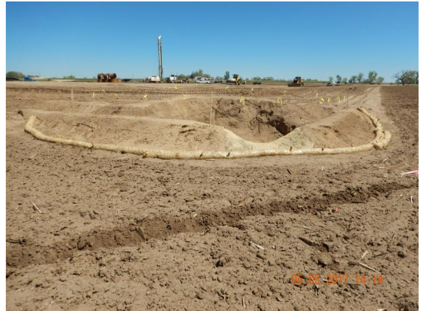
Photo 2. Photo taken from the northwest location, facing Southeast. A sediment trap has been installed with outlet protection devices.
