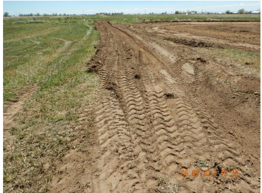
Photo 4. Photo taken May 5, 2017 from the eastern location, facing South. A ditch and berm BMP has been installed around the perimeter of the location. During the May 5, 2017 inspection, berm material did not appear consistently compacted throughout the location. Berm BMPs appeared to be further compacted during the May 11, 2017 inspection.
