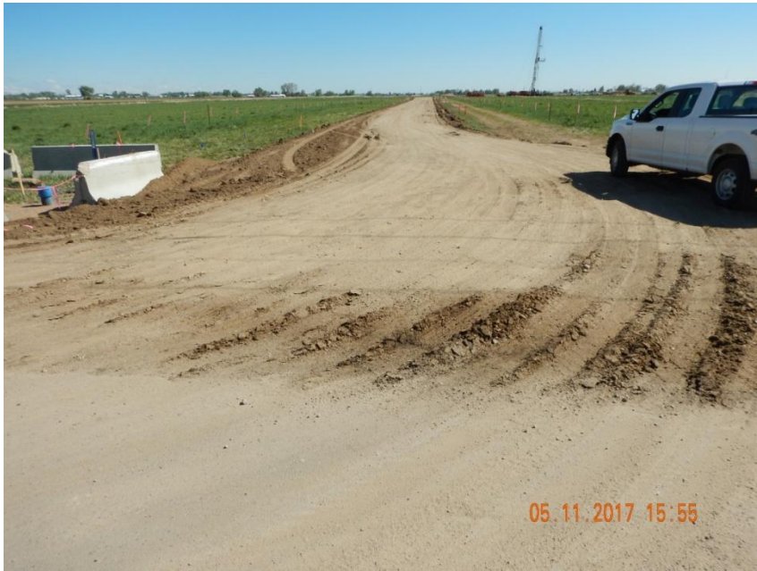
Photo 13. Photo taken May 11, 2017 from the entrance of location, facing South. Did not observe a tracking pad. COGCC staff contacted the Operator and the Operator communicated to COGCC staff that tracking pad material was supposed to be installed on that day. The Operator said street sweeping operations were being conducted.
