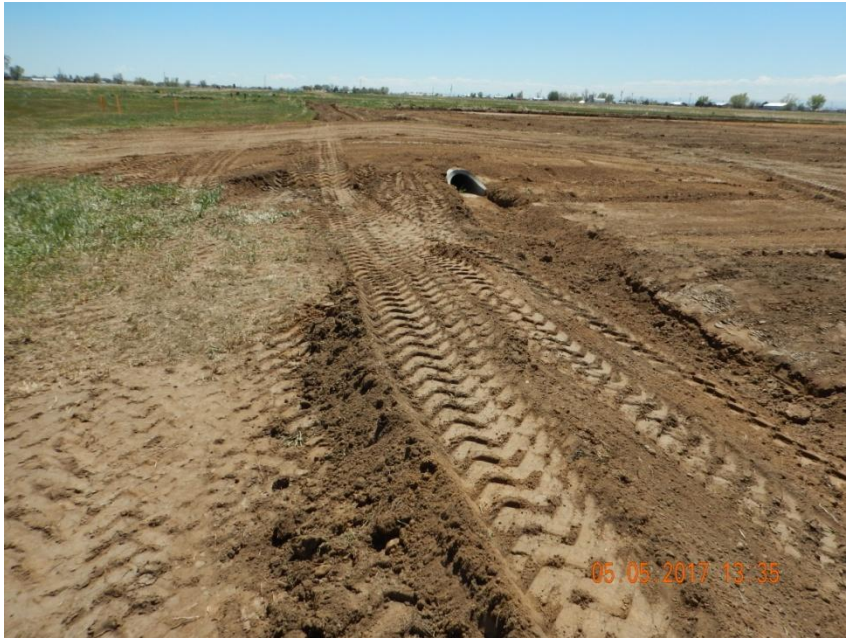
Photo 3. Photo taken May 5, 2017 from the eastern location, facing South. A ditch and berm BMP has been installed around the perimeter of the location. During the May 5, 2017 inspection, berm material did not appear consistently compacted throughout the location. Berm BMPs appeared to be further compacted during the May 11, 2017 inspection.
