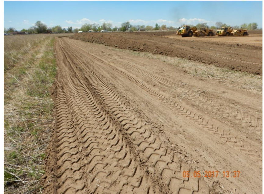
Photo 6. Photo taken May 5, 2017 from the southern location, facing West. A ditch and berm BMP has been installed around the perimeter of the location.
