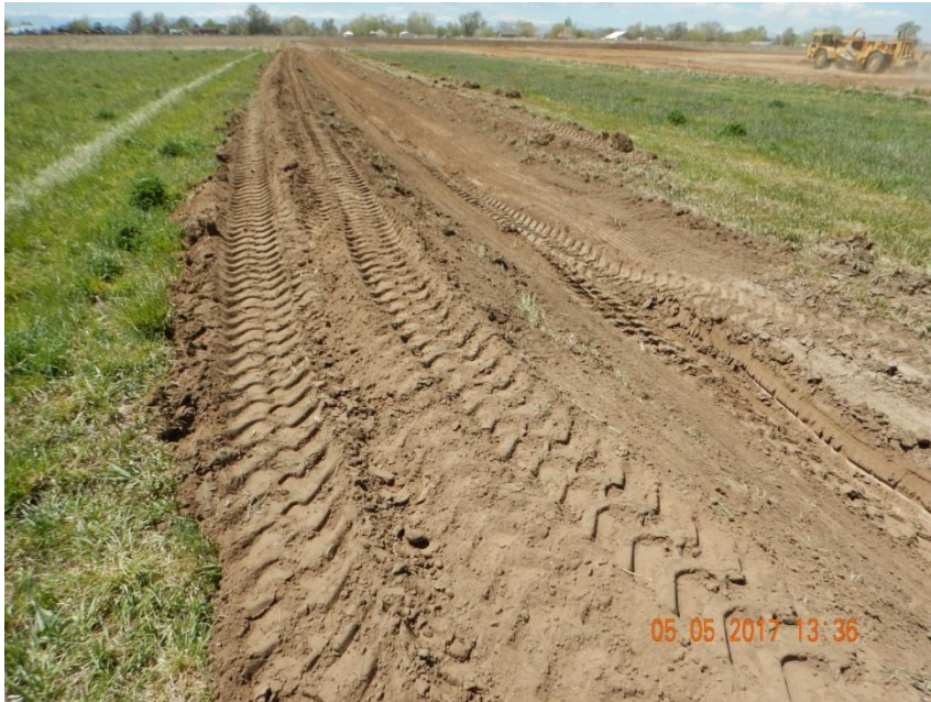
Photo 5. Photo taken May 5, 2017 from the southeastern location, facing West. A ditch and berm BMP has been installed around the perimeter of the location. During the May 5, 2017 inspection, berm material did not appear consistently compacted throughout the location. Berm BMPs appeared to be further compacted during the May 11, 2017 inspection.
