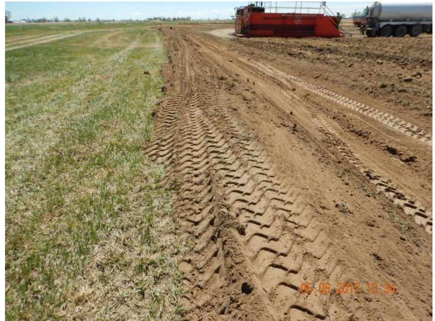
Photo 2. Photo taken May 5, 2017 from the northeastern location, facing South. A ditch and berm BMP has been installed around the perimeter of the location.
