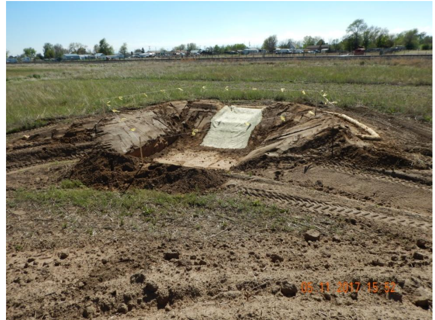
Photo 12. Photo taken May 11, 2017 from the southwest location, facing Southwest. A sediment trap has been installed with both outlet protection devices. Portions of the sediment trap berm do not appear consistently compacted.
