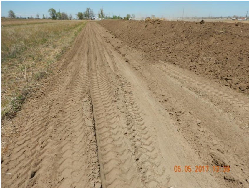
Photo 7. Photo taken May 5, 2017 from the western location, facing North. A ditch and berm BMP has been installed around the perimeter of the location. Topsoil stockpile has been salvaged and stored along the western location. Topsoil side slopes appear steep and may be difficult to stabilize.
