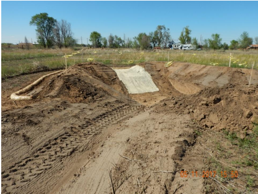
Photo 11. Photo taken May 11, 2017 from the northwest location, facing North. A sediment trap has been installed with both outlet protection devices. Portions of the sediment trap berm do not appear consistently compacted.
