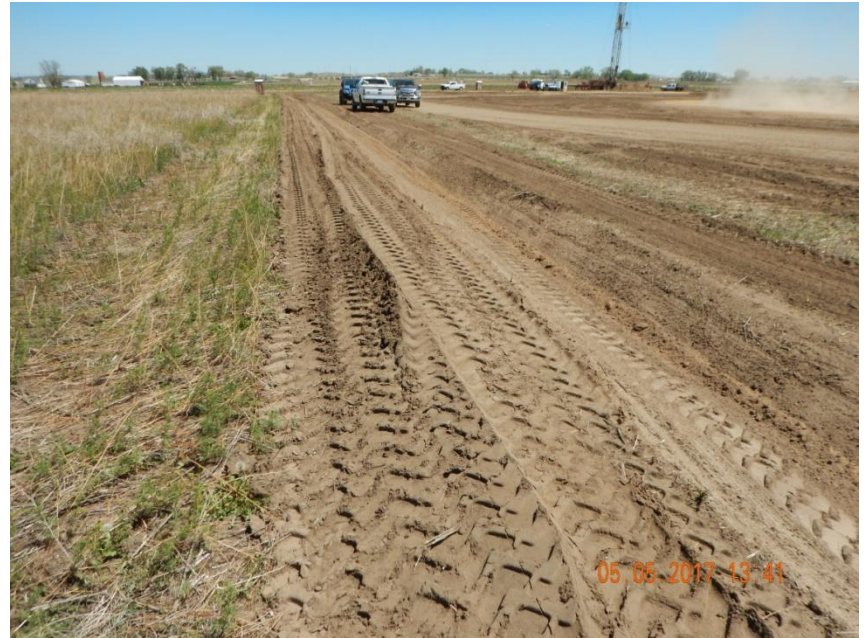
Photo 8. Photo taken May 5, 2017 from the northwestern location, facing East. A ditch and berm BMP has been installed around the perimeter of the location.
