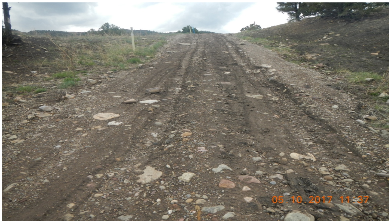
photo 1: Facing southwest along the access road. This portion of the access road has signs of vehicle rutting .
