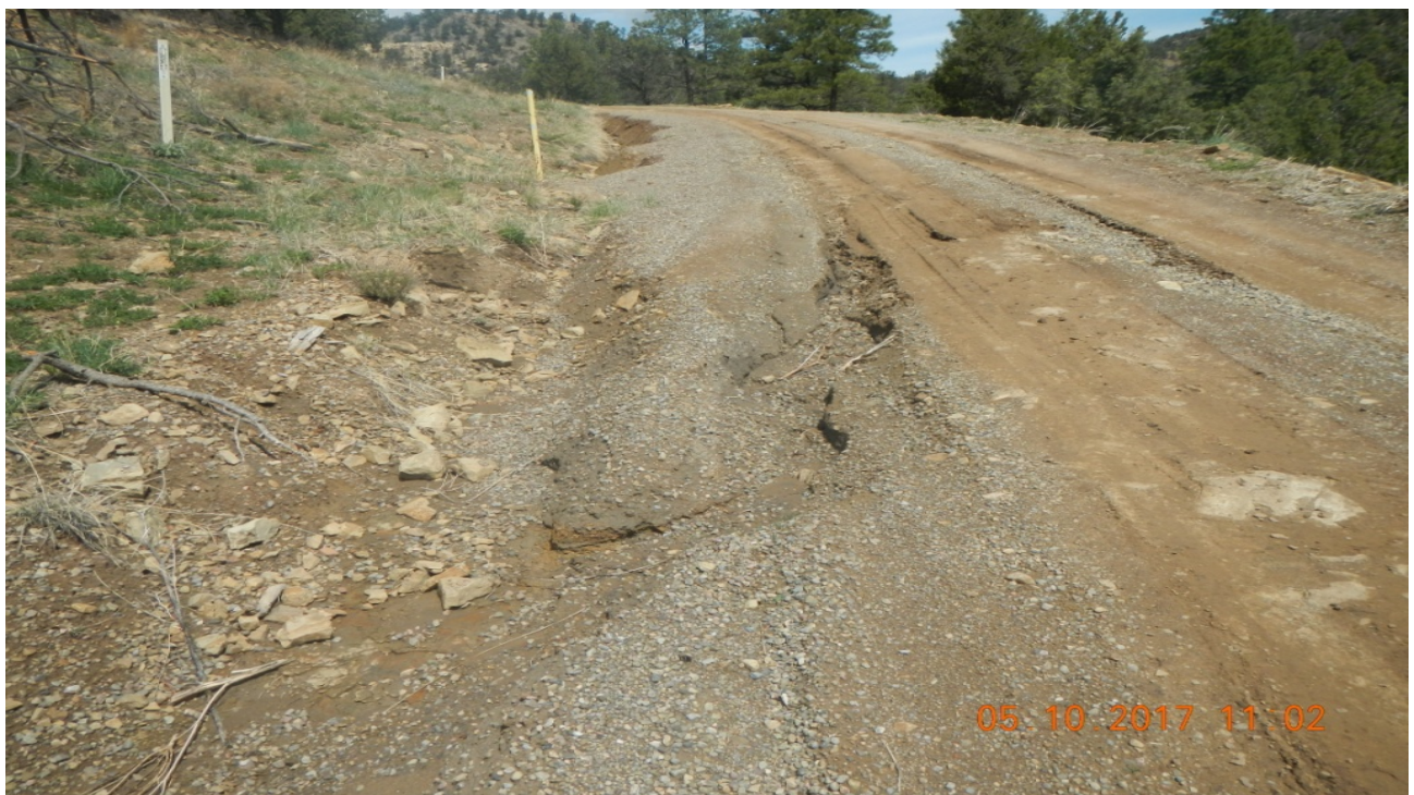
photo 2: There are signs of erosion in areas of the main road.
