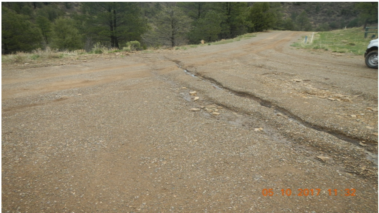
photo 4: Stormwater from the above photo is causing erosion across the main road.
