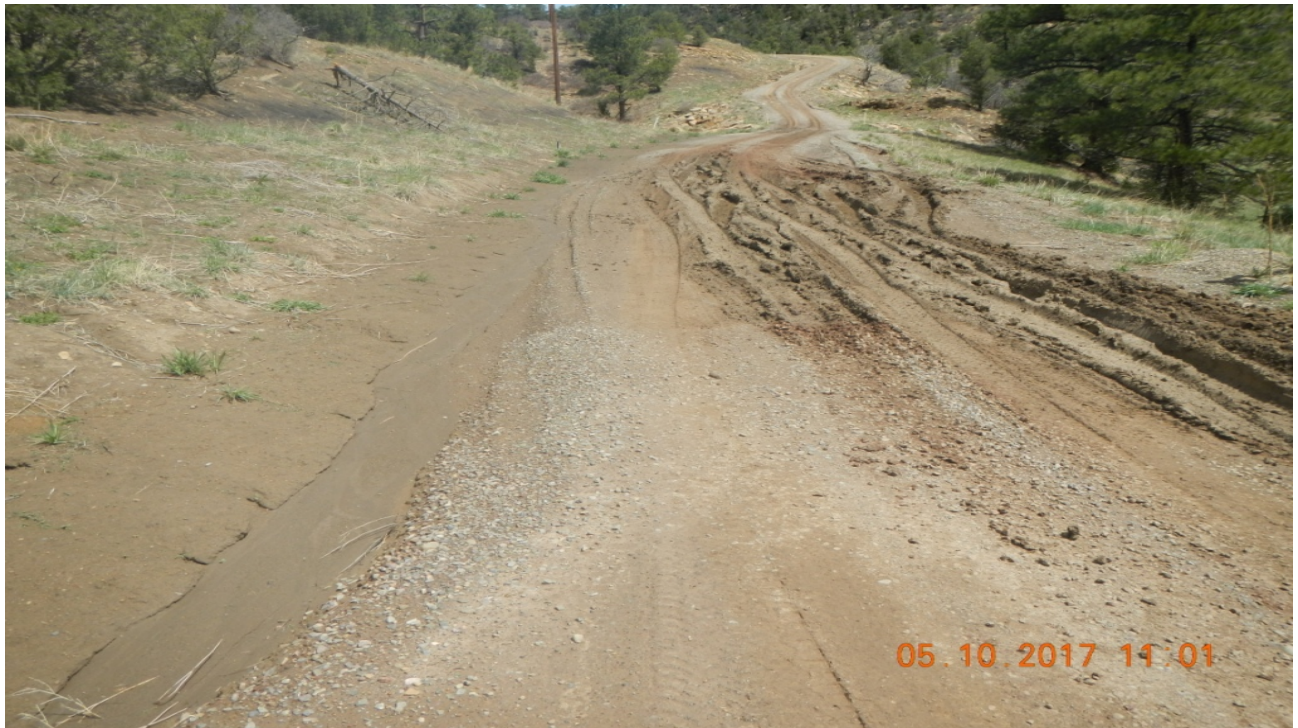
photo 1: Facing northeast along the main access road. There is vehicle rutting in this area of the road.
