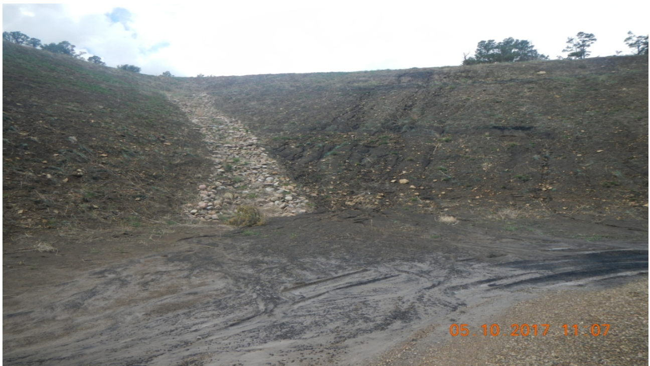
photo 6: There are signs of erosion occurring at the southwest corner of the pad which is depositing sediment to this area.
