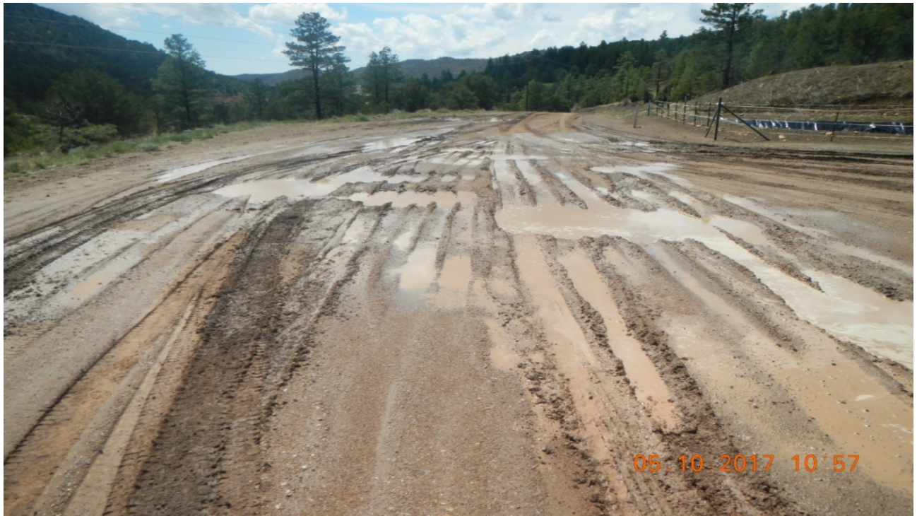
photo 3: Facing south along the main road which goes thru the location. There is vehicle rutting and potholes in this area of the road.
