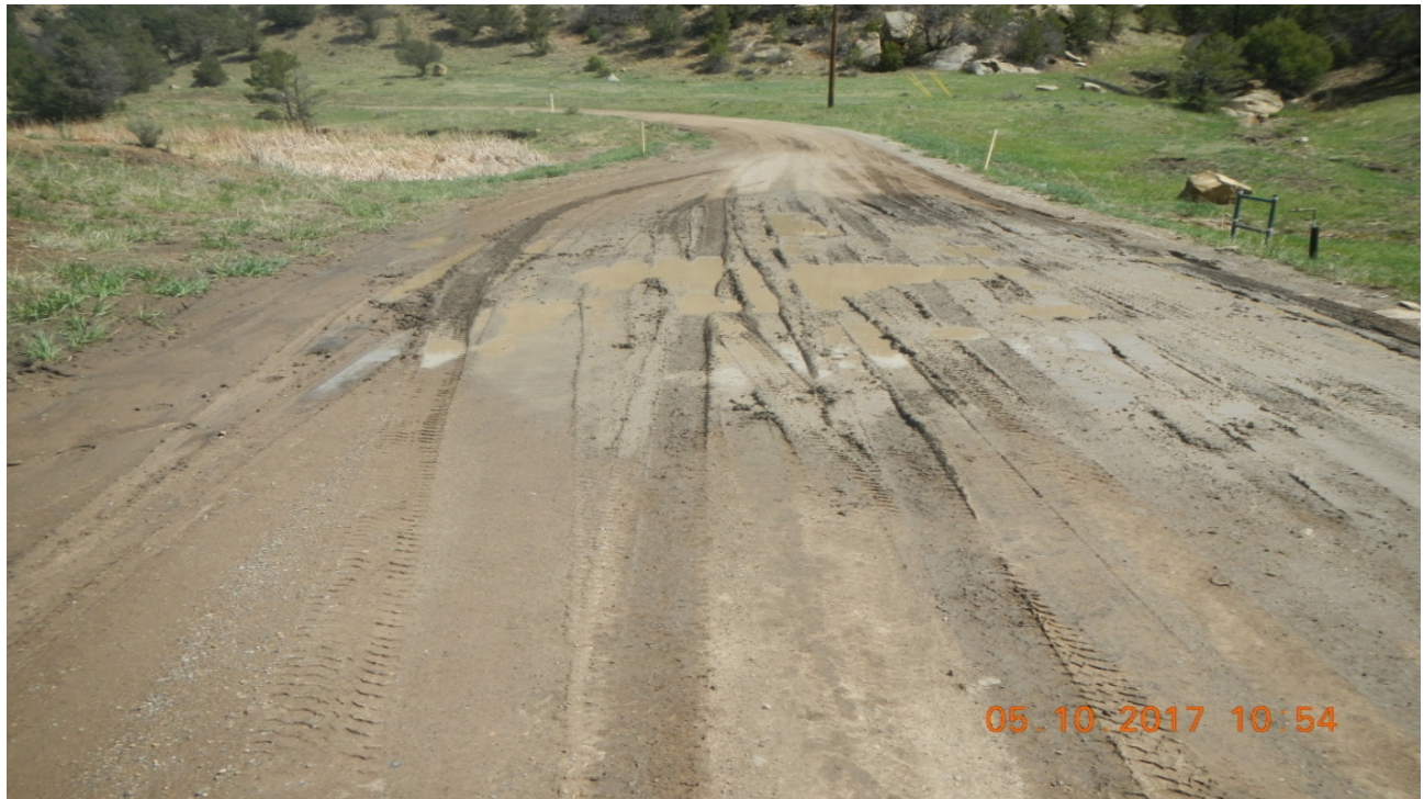
photo 1: Facing northeast along the main access road. There is vehicle rutting and potholes in this area of the road.
