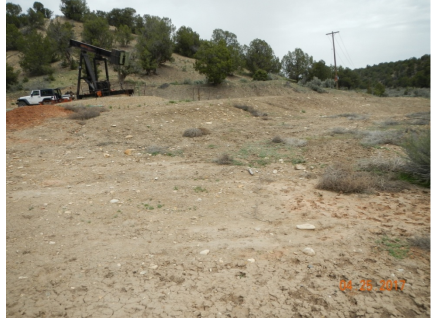
Photo 6: View of the southwestern edge facing eastward. Erosional channels are forming all along the southern edge.
