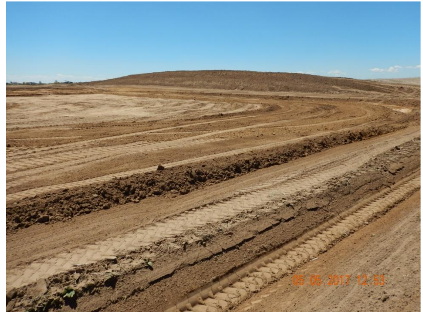
Photo 4. Photo taken from the northwestern location, facing West. Topsoil has been salvaged and stored along the western perimeter of the location.
