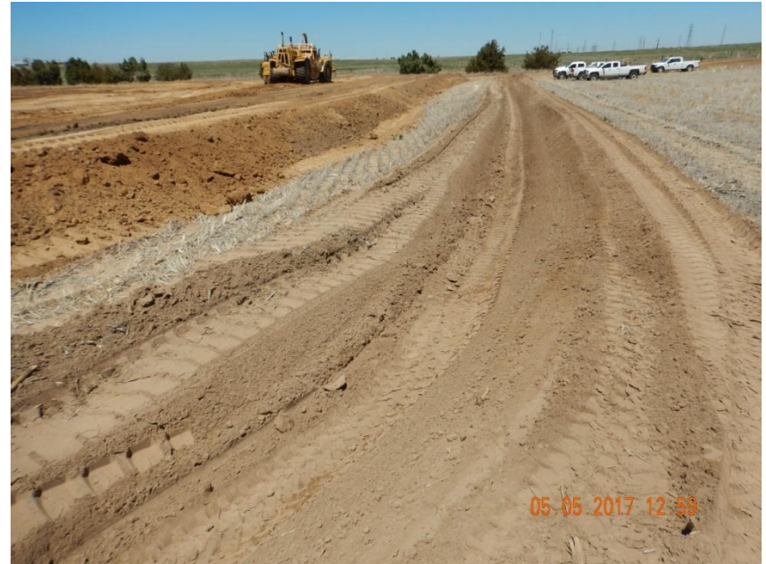
Photo 8. Photo taken from the southeastern location, facing North. A ditch and berm BMP has been installed around the entire perimeter of the location.
