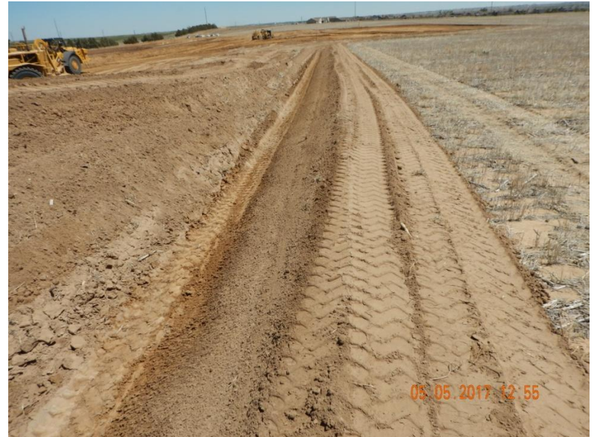
Photo 6. Photo taken from the southwestern location, facing East. A ditch and berm BMP has been installed around the entire perimeter of the location.
