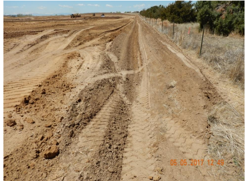
Photo 2. Photo taken from the northeast location, facing West. A ditch and berm BMP has been installed around the entire perimeter of the location.
