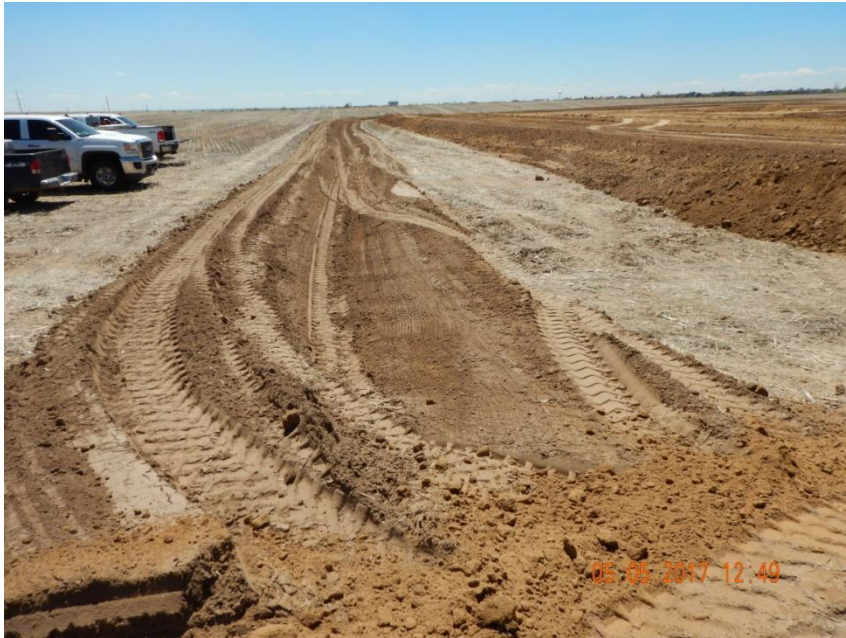
Photo 1. Photo taken from the northeast location, facing South. A ditch and berm BMP has been installed around the entire perimeter of the location.
