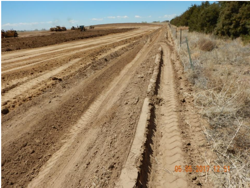
Photo 3. Photo taken from the northern location, facing West. A ditch and berm BMP has been installed around the entire perimeter of the location.
