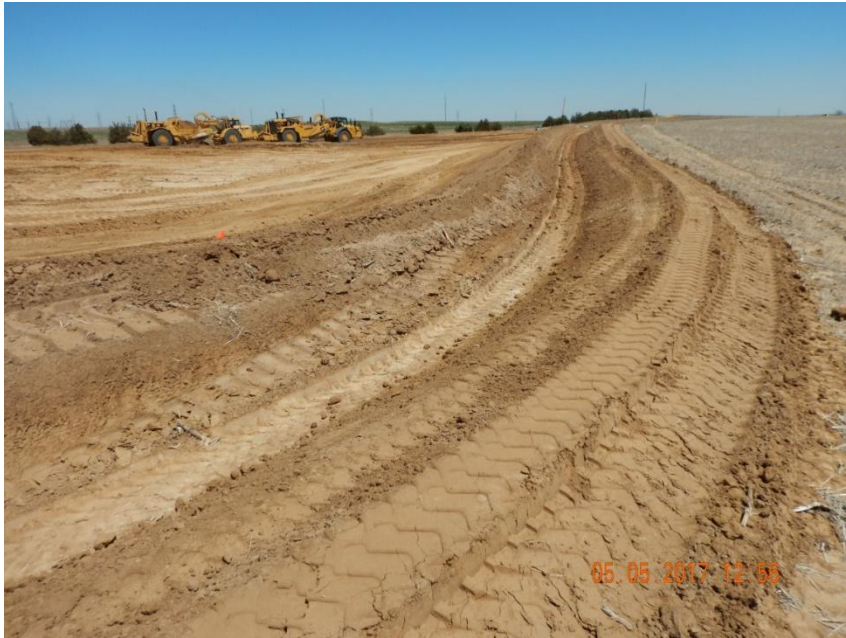
Photo 7. Photo taken from the southern location, facing East. A ditch and berm BMP has been installed around the entire perimeter of the location.
