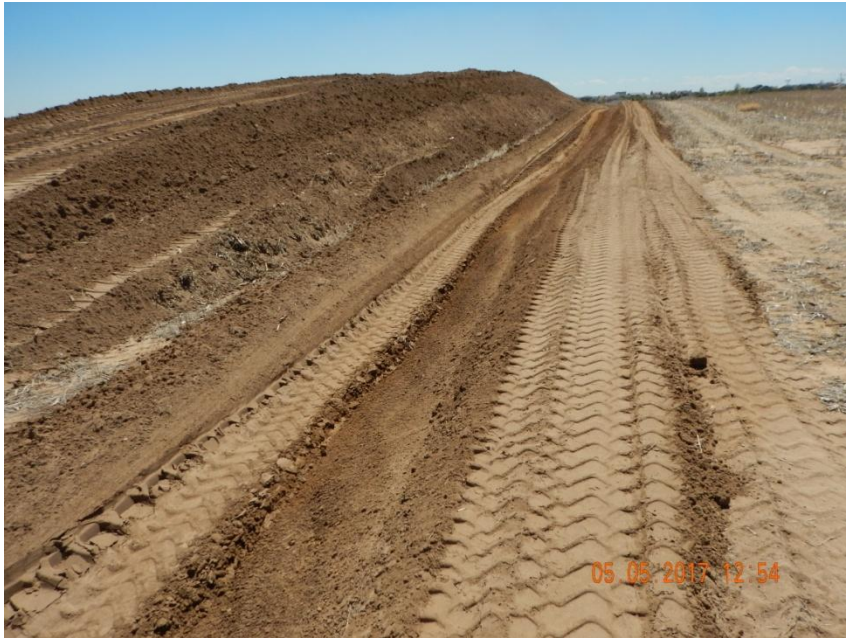
Photo 5. Photo taken from the western location, facing South. A ditch and berm BMP has been installed around the entire perimeter of the location.
