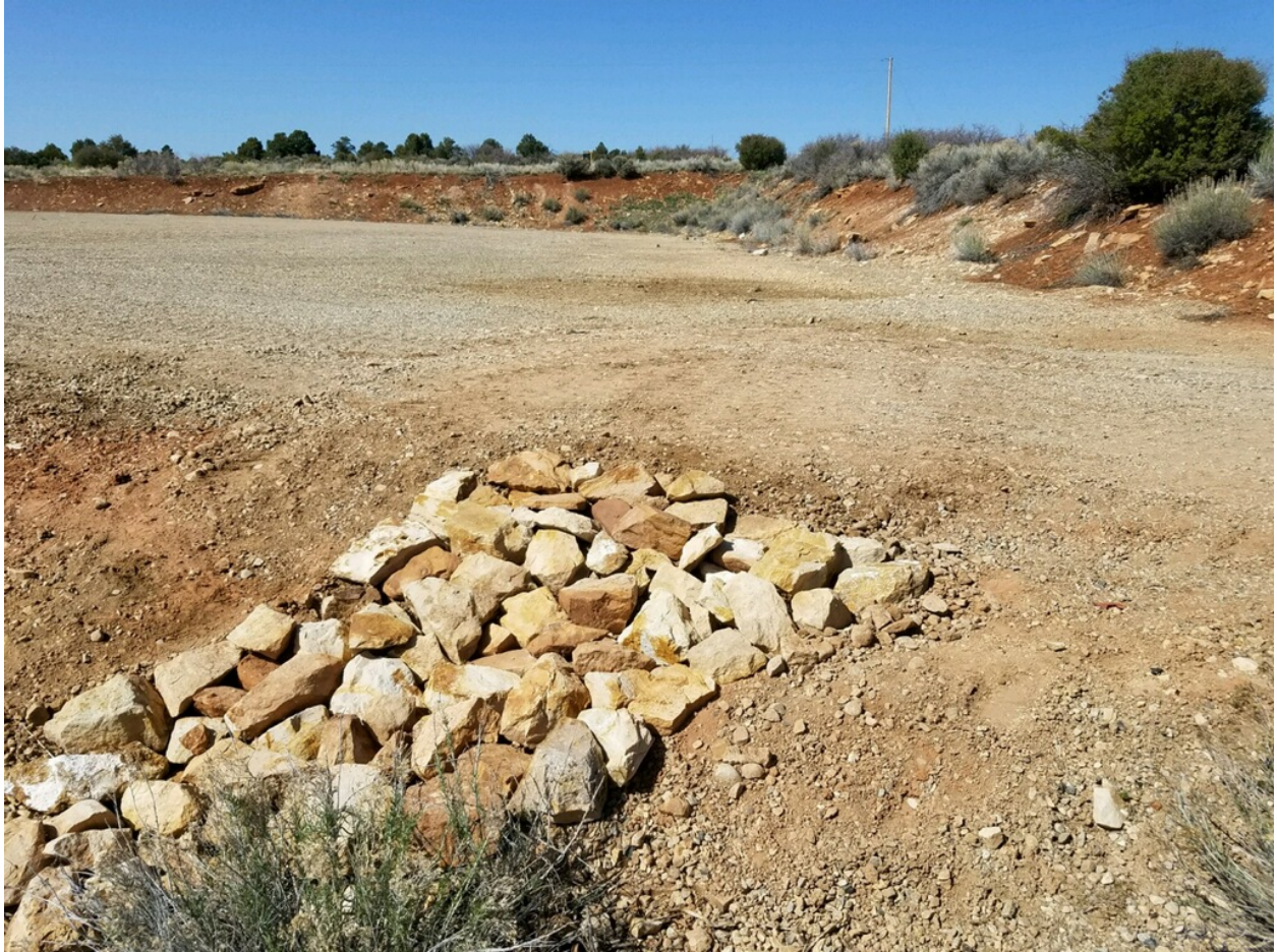
Photo 1: Repaired erosion on well pad/gravel area. Installed rip-rap rundown on slope for additional stabilization.
