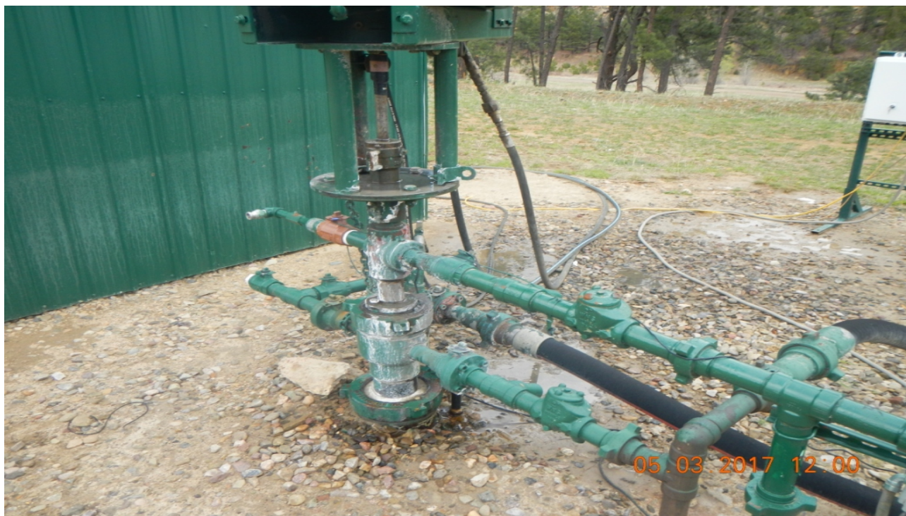
photo 2: There is a slow dripping water leak coming out of the wellhead.
