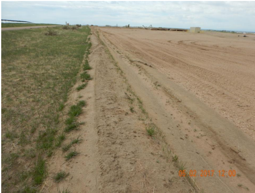
Photo 1. Photo taken from the eastern perimeter of the location, facing South. Ditch and berm BMP has been installed around most of the location in conjunction with other BMPs and appears to be properly functioning.
