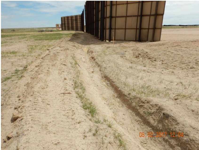
Photo 7. Photo taken from the northwest perimeter of the location, facing East. Ditch and berm BMP has been installed along portions of the northern perimeter of the location.
