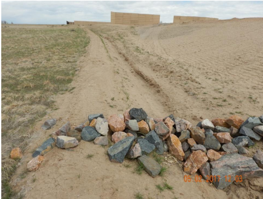
Photo 5. Photo taken from the southwestern perimeter of the location, facing North. Ditch and berm BMP has been installed in conjunction with check dams prior to the sediment trap.
