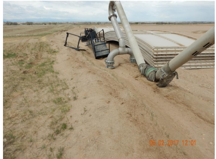
Photo 2. Photo taken from the southern perimeter of the location, facing West. Oil and gas locations are to be kept free of supplies. Appears supplies are being stored along the southern location, some of which have been placed along the BMP area.
