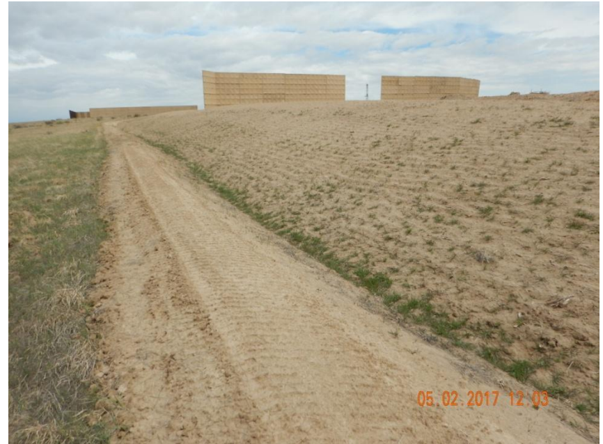
Photo 6. Photo taken from the western perimeter of the location, facing North. Ditch and berm BMP has been installed around the topsoil stockpile. Topsoil has been salvaged, stored and temporarily stabilized along the western perimeter of the location.
