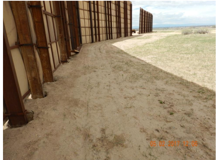
Photo 8. Photo taken from the northeastern perimeter of the location, facing West. No stormwater BMP observed. Operators do need to control run-on onto location to minimize erosion and site degradation which may require stormwater BMPs.
