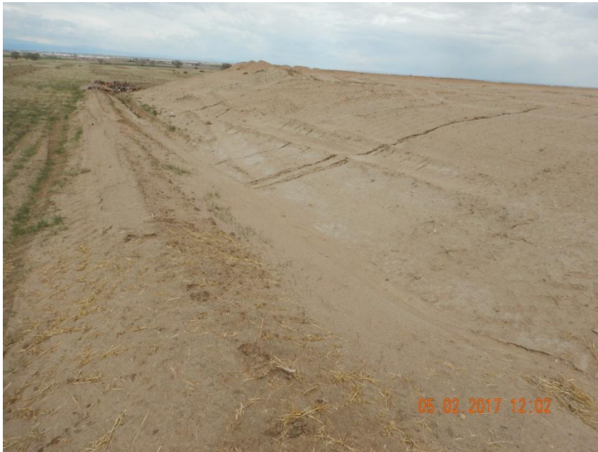
Photo 3. Photo taken from the southwestern perimeter of the location, facing West. Minor rill erosion along the fill slope. BMPs are in place to capture sediment laden storm runoff from leaving location.
