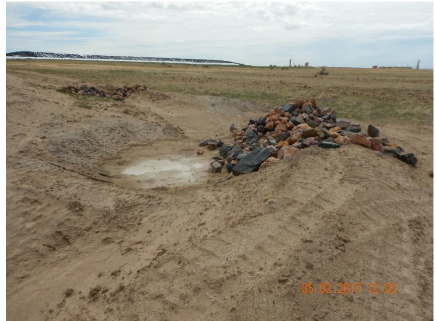
Photo 4. Photo taken from the southwest perimeter of the location, facing Southeast. Sediment trap has been installed with both inlet and outlet protection, as well as check dams.
