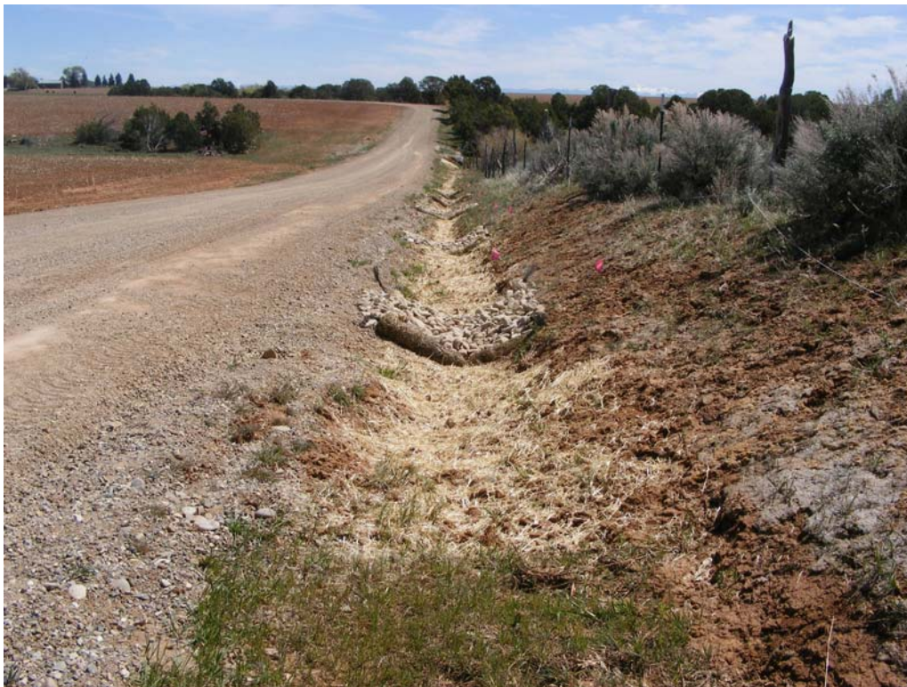
Photo 2: Control measure improvements to control ditch cutting have been installed on CX-7 access road.
