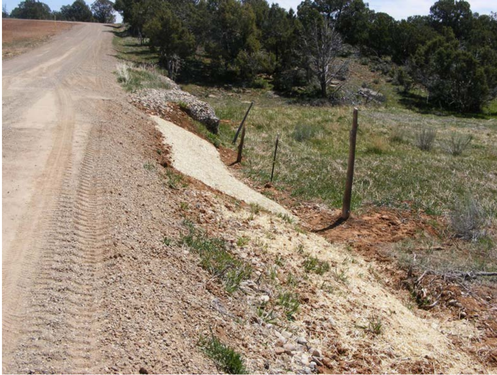
Photo 3: Slope has been re-seeded and blanketed on CX-7 access road.
