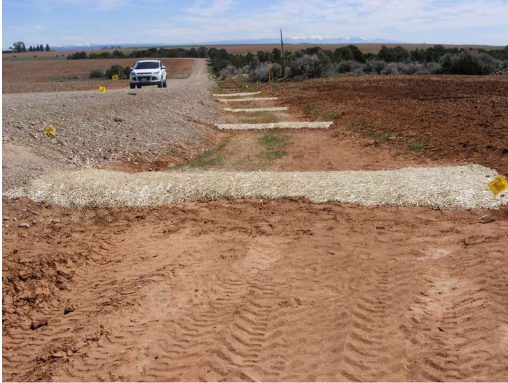
Photo 1: Control measure improvements installed adjacent to farm field and CX-7 access road. Swales and ditch have been re-seeded.
