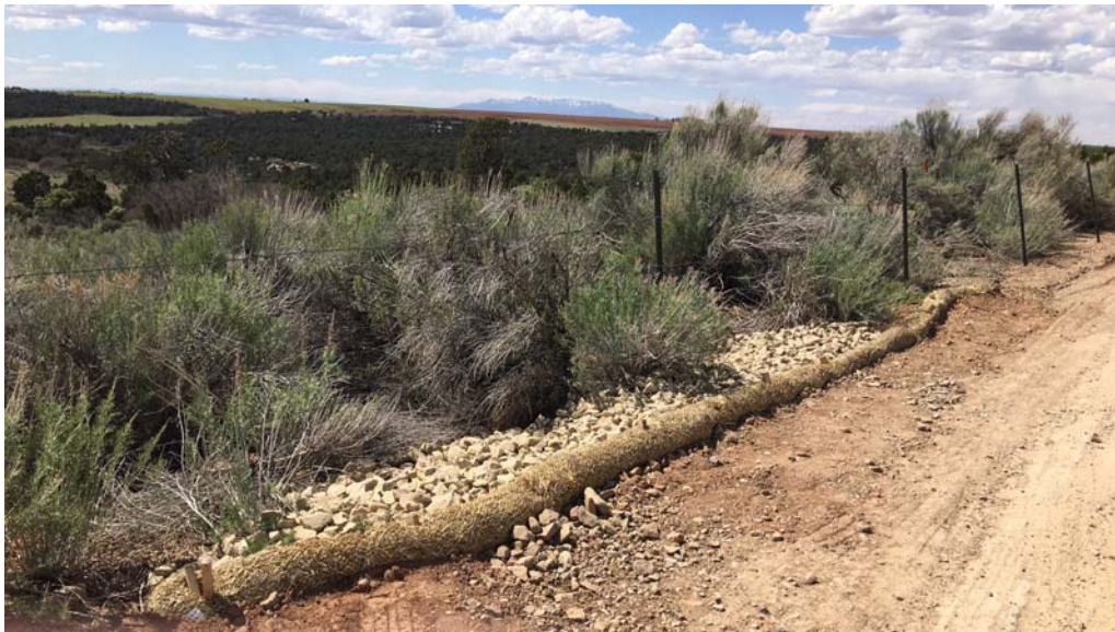
Photo 2: Control measures installed to prevent future erosion.
