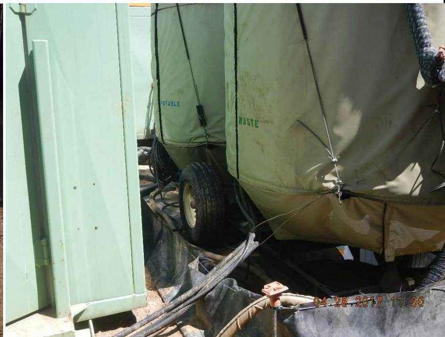
Secondary Containment – Potable Water and Waste
