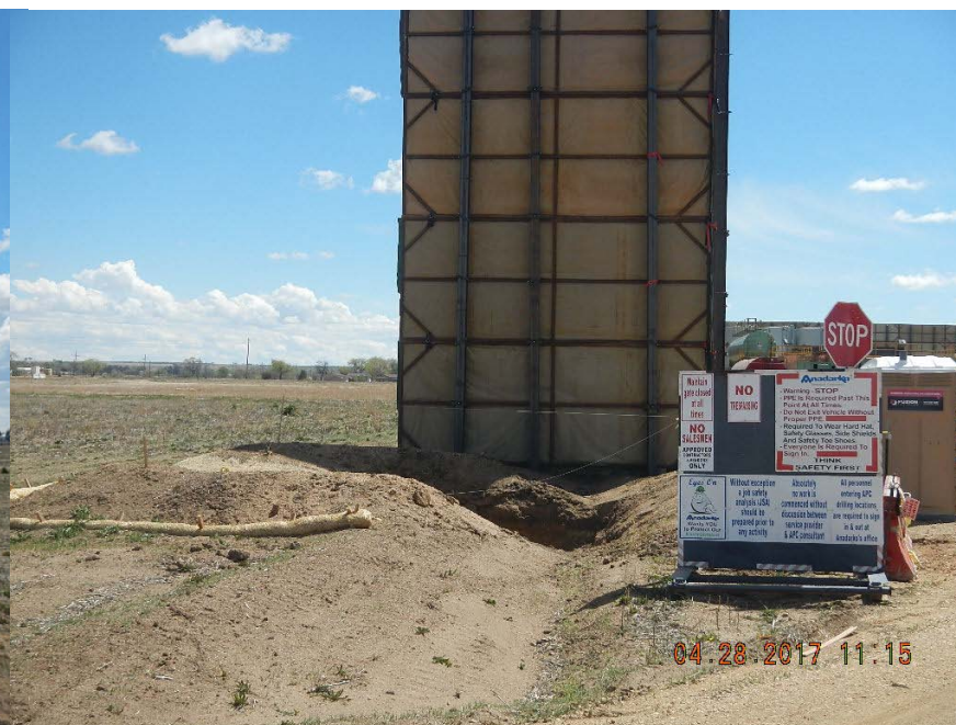
Stormwater BMP, Retention and Waddles at Entrance
