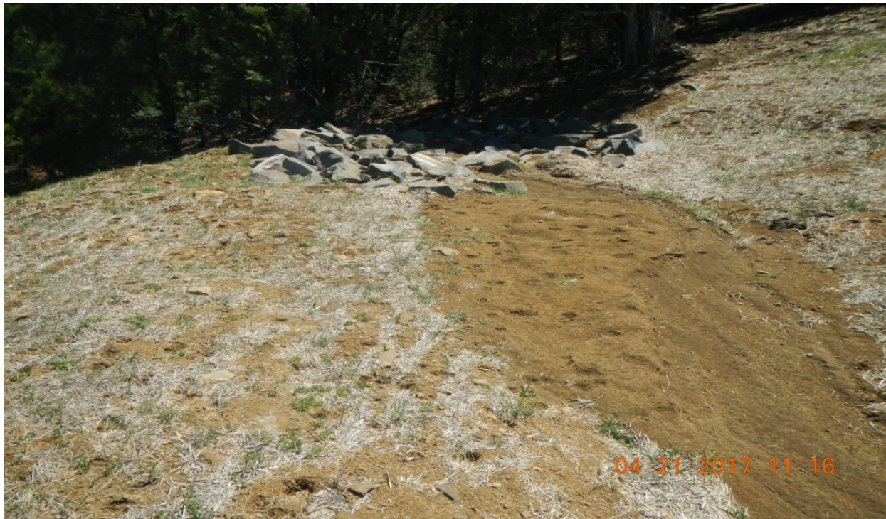
photo 7: The stormwater is directed to this point at the east side of the location. Sediment is accumulating in front of the rock rip-rap.
